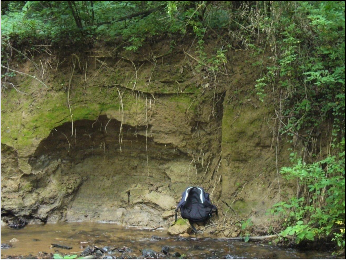
Figure 5: An actively eroding stream bank directly upstream from a breached mill dam on Little Piney Run.
