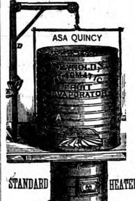
A Round Trays, as they appear in operation, B, Automatic Hot Air Governor or Circula-tor; C, Standard Furnace; D. E. Crane for raising or removing all or any number of Trays off or over the Heater, as desired. The position of the Fruit over the Her
