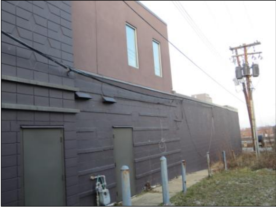
Figure 12. 5321 1 st Place, NE, south wall, radio transmission station (center), encapsulated by WOOK-TV (foreground); a later addition (rear), and a second story addition, view north (Source: Jennifer Sparenberg, 2013)
