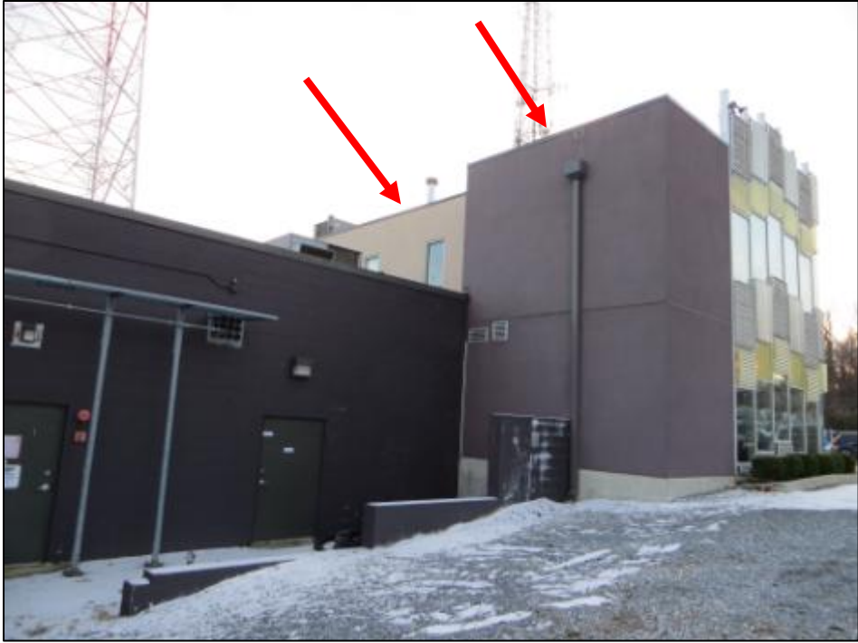
Figure 20. 5321 1 st Place, 2007 additions identified by red arrows, view west (Source: Jennifer Sparenberg, 2013)
