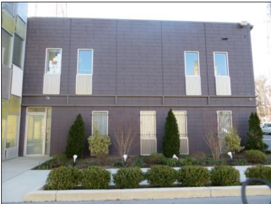
Figure 17. 5321 1 st Place, NE, side entry door on north wall, 2007 addition visible on left, view south (Source: Jennifer Sparenberg, 2013)
