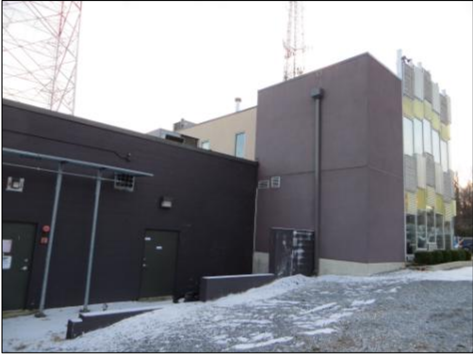
Figure 18. 5321 1 st Place, NE, addition (left) constructed circa 1963-1974, two story addition constructed in 2007 (right), north wall, view south (Source: Jennifer Sparenberg, 2013)
