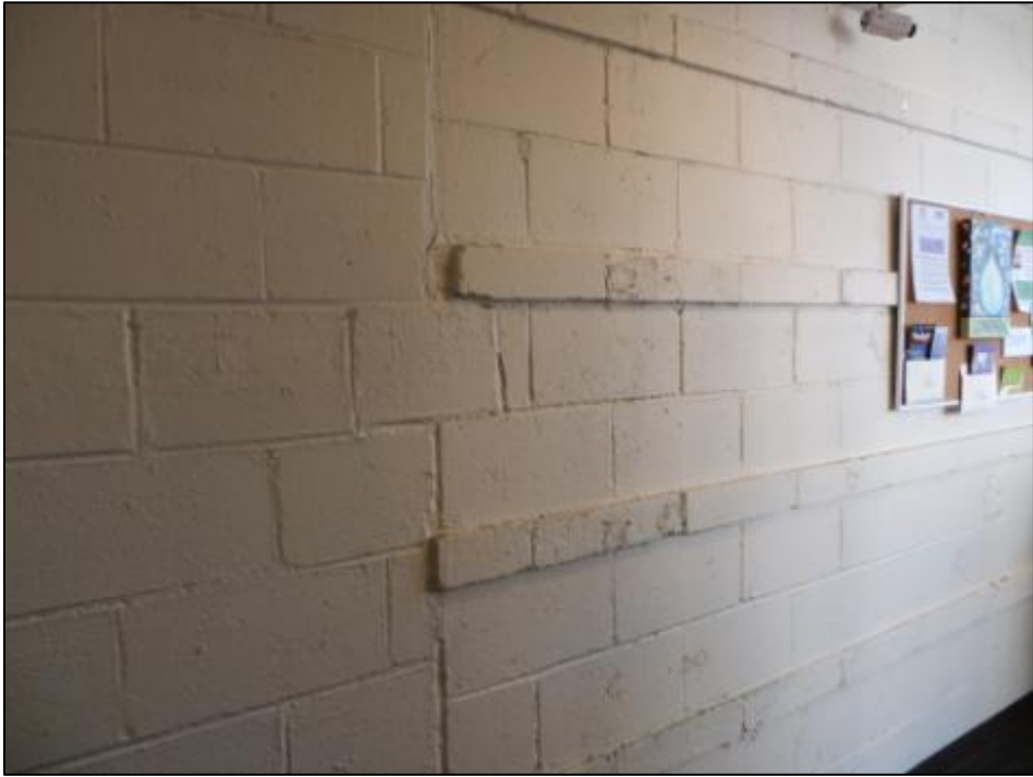
Figure 13. 5321 1 st Place, NE, north exterior wall of radio transmission station (Source: Jennifer Sparenberg, 2013)
