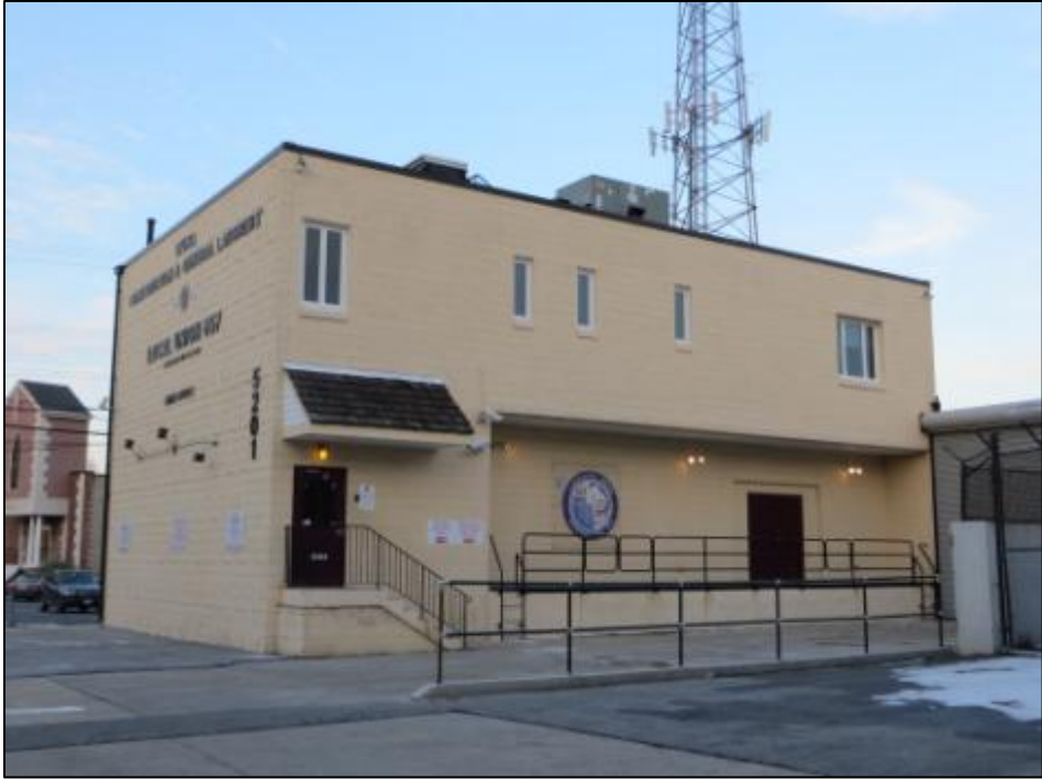
Figure 4. 5201 1 st Place, NE, view north (Source: Jennifer Sparenberg, 2013)
