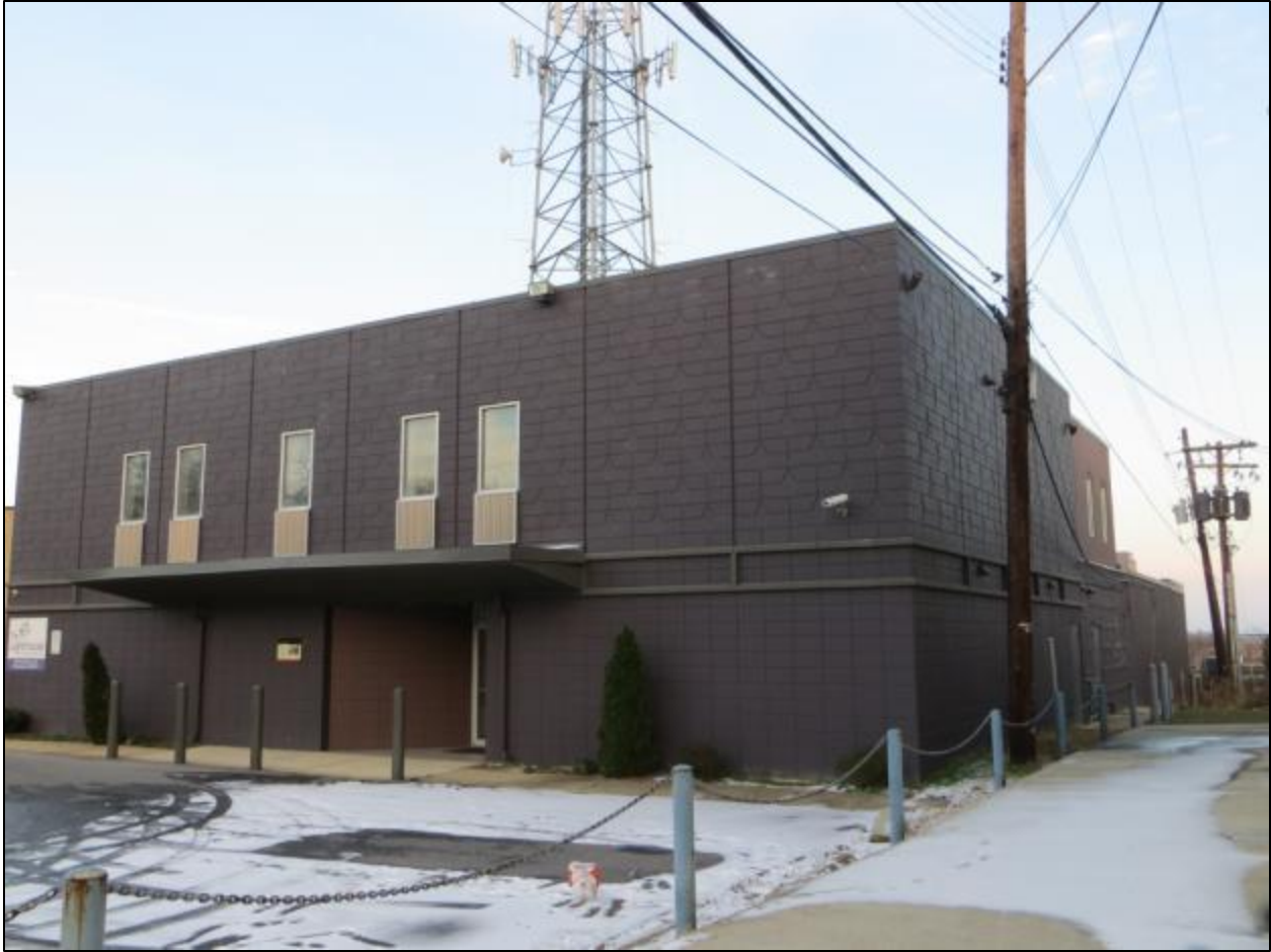
Figure 3. 5321 1 st Place, NE, Front and south façades, view east, note transmission tower behind building (Source: Jennifer Sparenberg, 2013)
