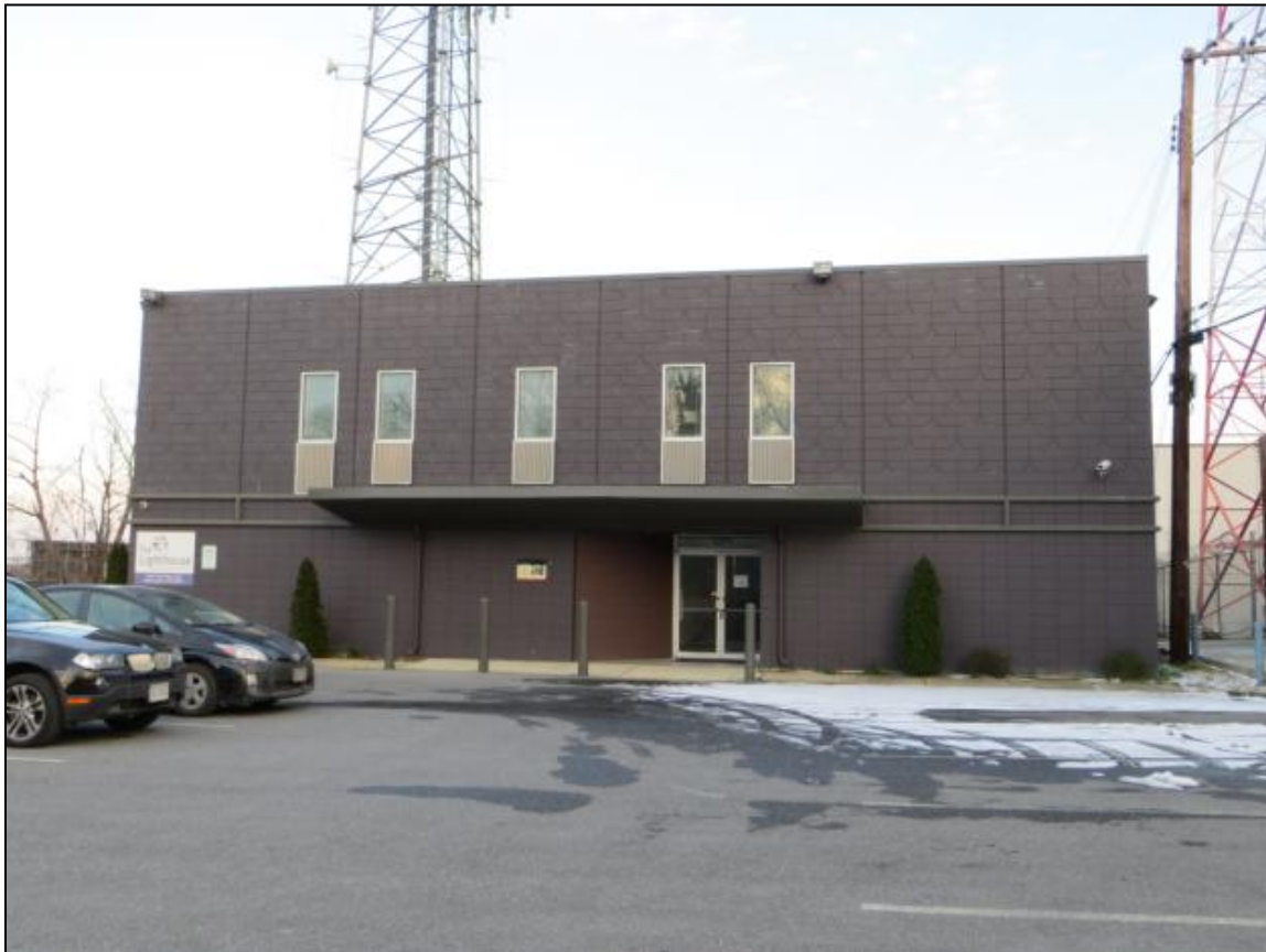
Figure 22. 5321 1 st Place, NE as it appeared in February 2013. Note: 2007 additions not visible in photograph (Source: Jennifer Sparenberg, 2013)
