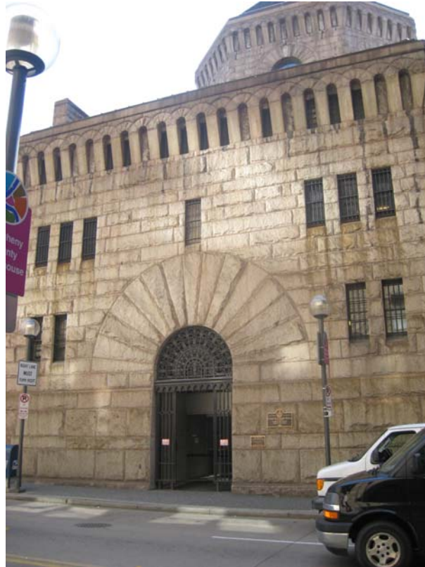
Figure 2: Allegheny County Jail, Ross Street entrance [Photograph by author]
