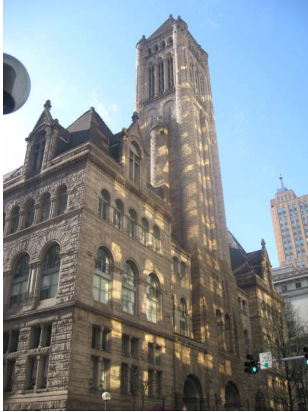
Figure 1: Allegheny County Courthouse [Photograph by author]
