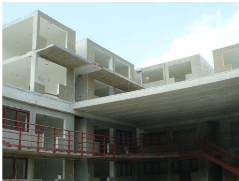
Figure 32: Precast concrete modular cells, with balconies, produced by Oldcastle Precast [Oldcastle Precast] 141
