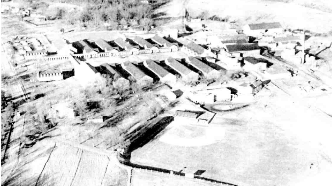
Figure 26: The Workhouse, as viewed from the air, circa 1960 [Courtesy of the Workhouse Museum]
