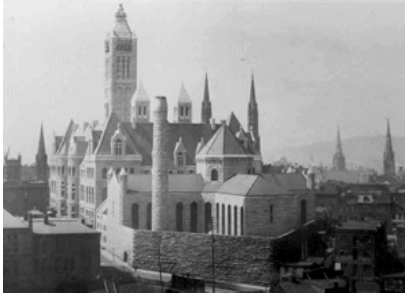
Figure 4: Allegheny Courthouse and Jail, undated [Allegheny County]
