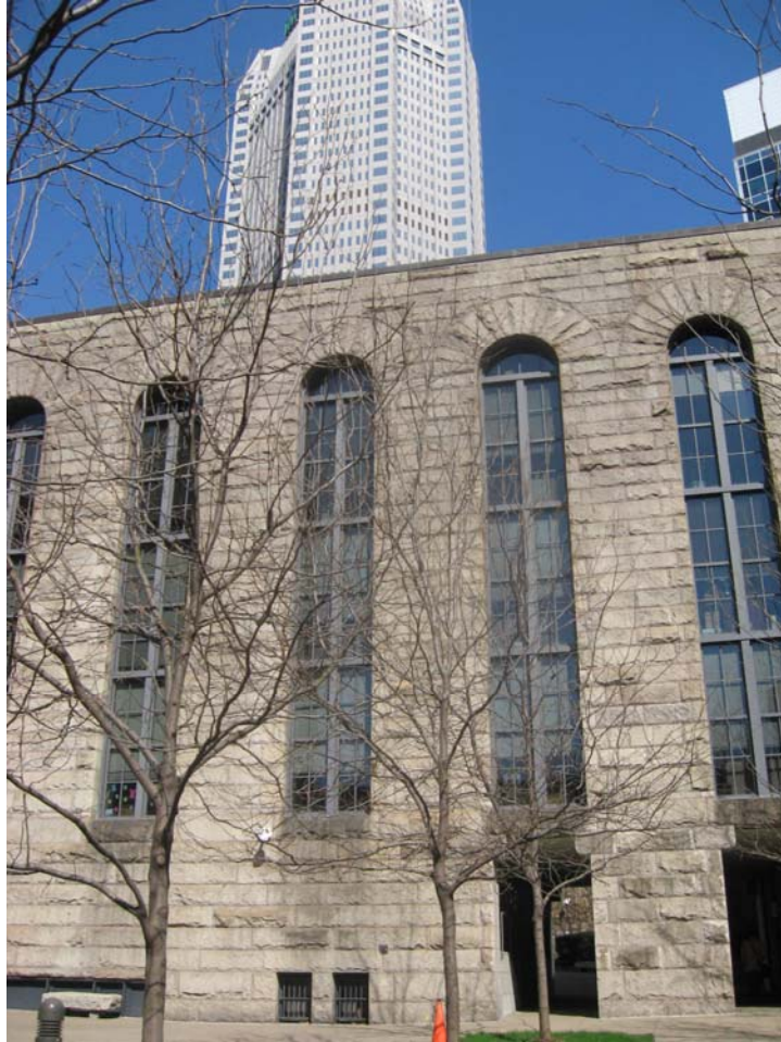
Figure 6: Aluminum windows, with faux double-hung sash, replacing Richardson's original wood windows. [Photograph by author]
