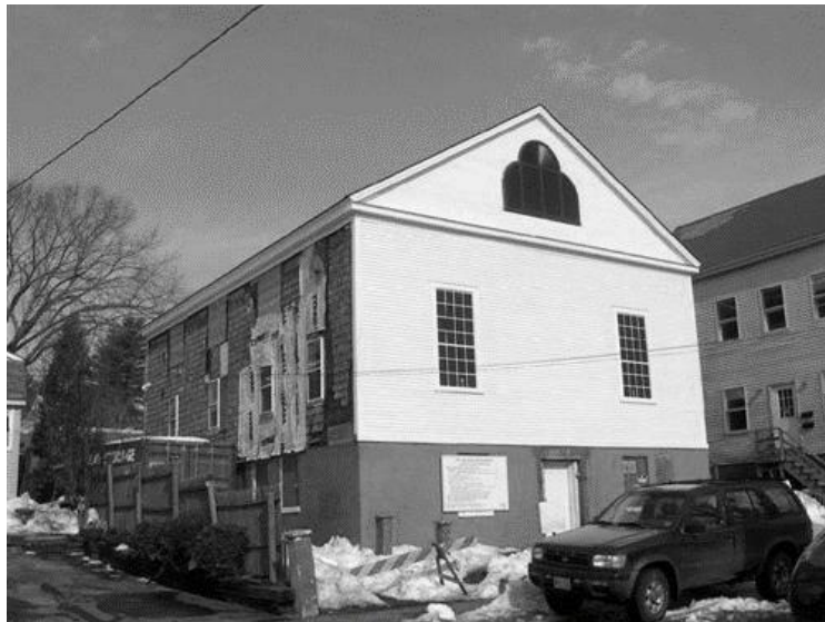
Figure 7. Abyssinian Meeting House, Portland, Maine [Abyssinian Restoration Project, 2011].
