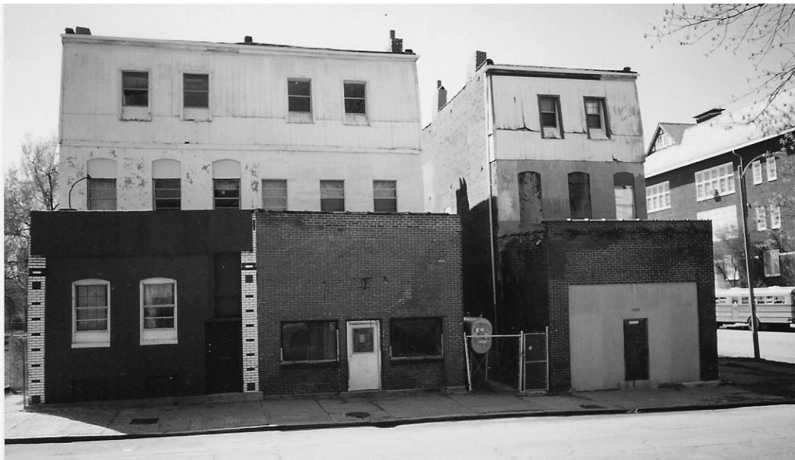
Figure 14. Tillie's Corner pre-collapse [Courtesy of Carla Alexander, 2002]
