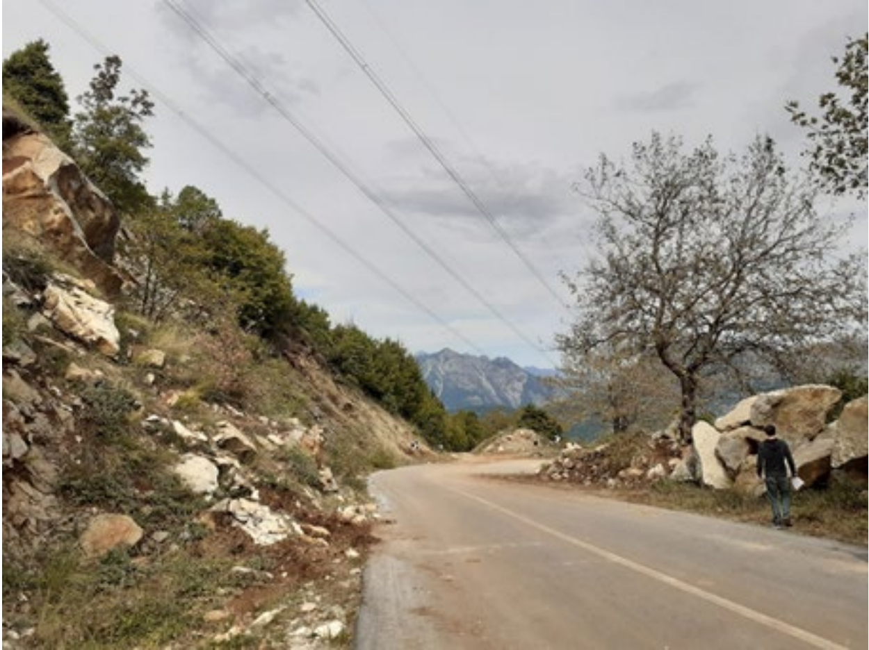
Figure 6.35. Planar sliding and rockfalls in limestone rockmass. Road to Oxia. (39.3895330°N, 21.6145240°E)
