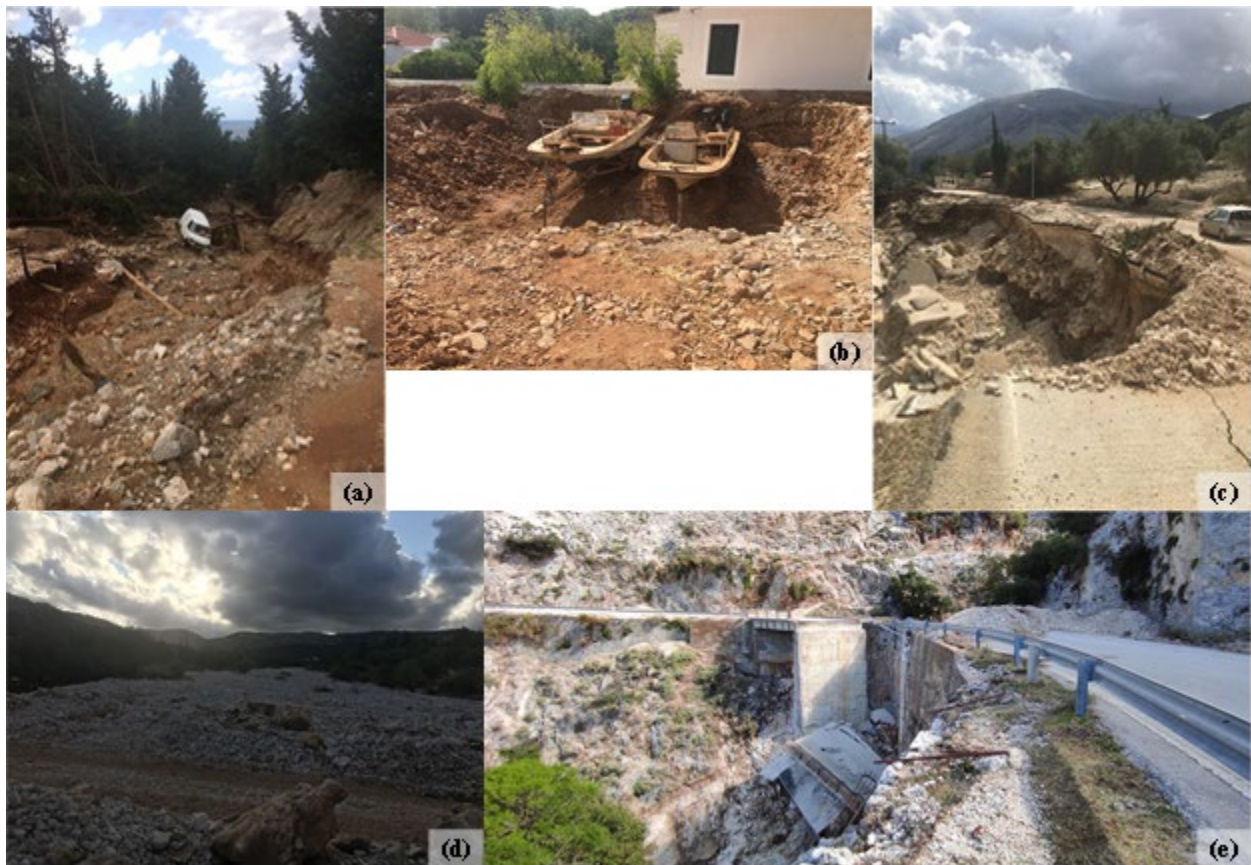
Figure 4.6. Characteristic damages in Cephalonia island following Medicane Ianos: a) Riverbank Erosion, b) debris flow within a rural community, c) road embankment failure, d) extensive debris flow, e) bridge collapse.
