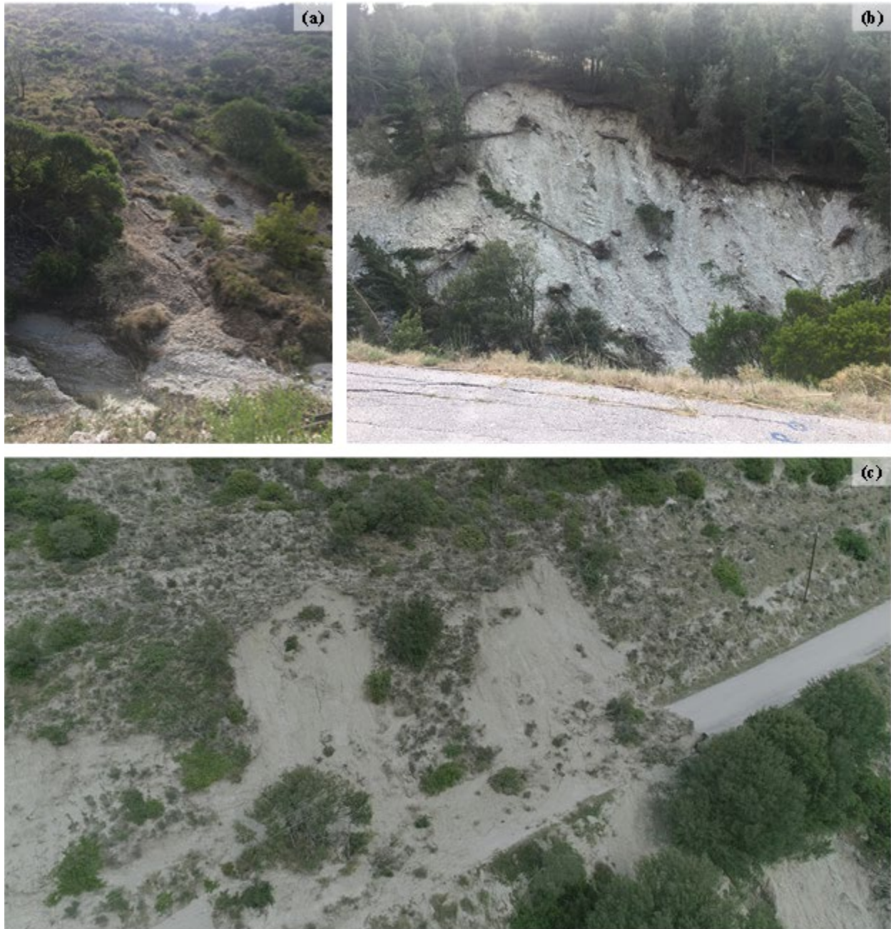
Figure 6.2. Rotational slides along the road to Myrtos beach through Divarata village: a) 38.33571944°N, 20.543633°E; b) 38.3365027°N, 20.5427166°E, c) 38.337106°N, 20.541785°E
