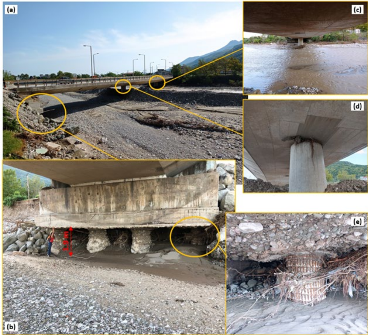
Figure 5.15. Photos of Bridge No. 7, the road bridge crossing Pamissos river in the center of Mouzaki (39.427341667°N; 21.667275000°E): (a) side view; (b) abutment scour; (c) unaffected, opposite (SE) side; (d) debris stuck within the connection between pier and deck indicating flood water height.
