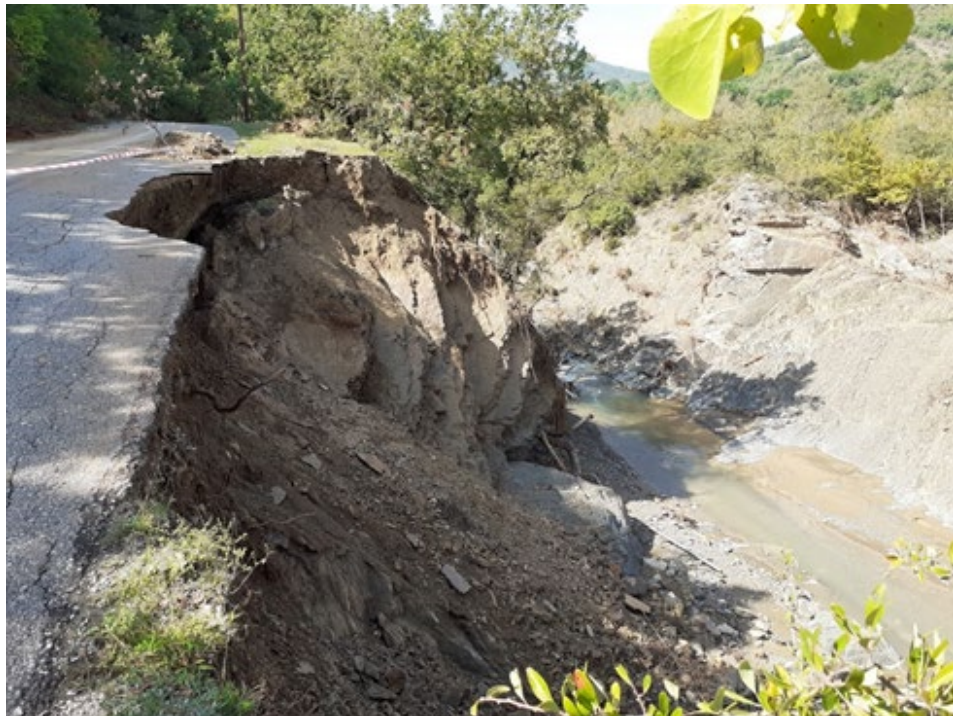
Figure 7.25. Riverbank erosion – slope failure that partially damaged the road (39.2515460°N, 21.8736180°E).
