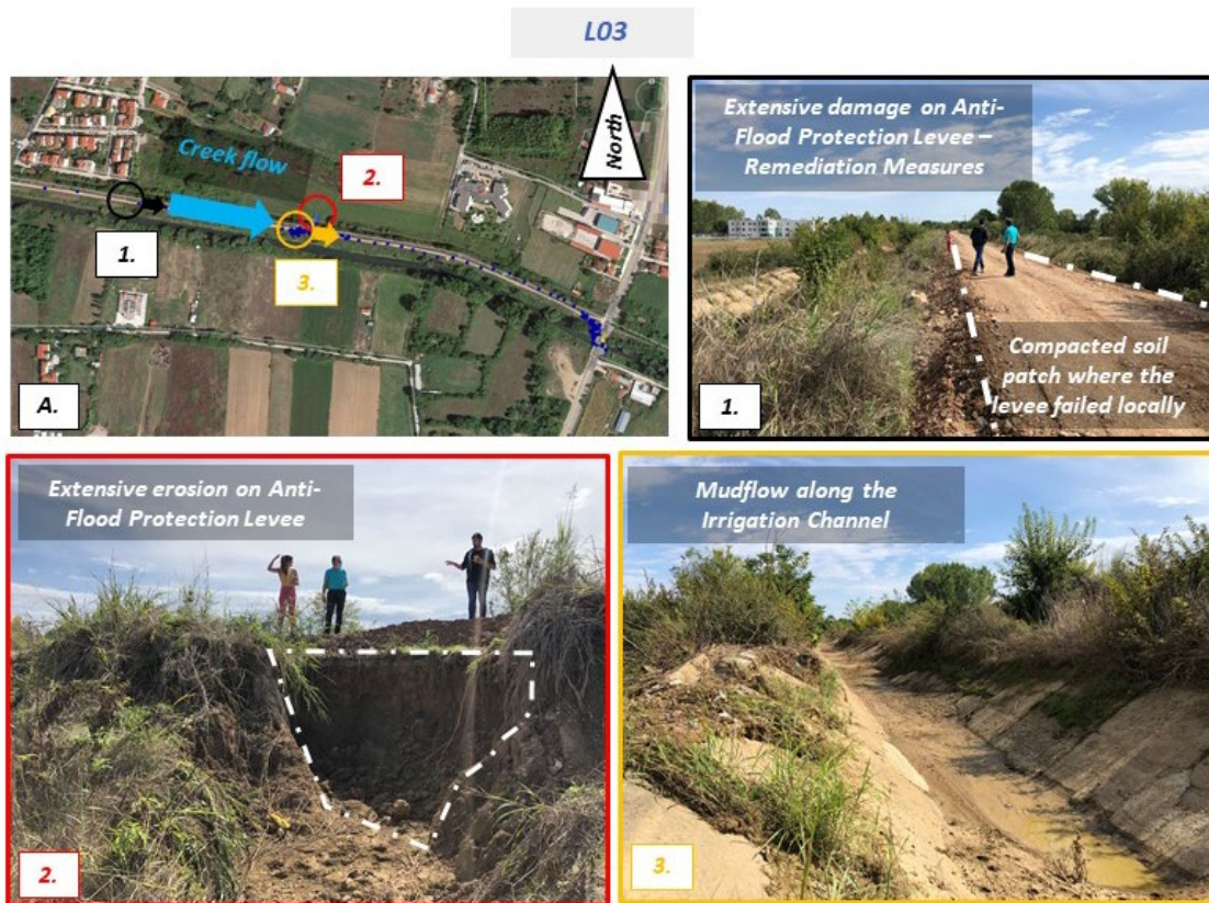
Figure 8.8. (A) location of Flood Protection Levee 03 (39.348173°N; 21.915506°E); (1) extensive damage with loss of a significant part of the levee section (was compacted when we arrived there on October 2, 2020); (2) extensive erosion caused most probably by vortices of the flooded irrigation channel; (3) debris build up on the irrigation channel (photo looking downstream).
