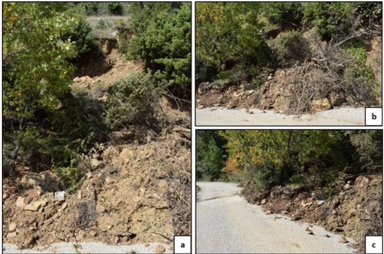
Figure 6.15. Rotational slide on the road to Oxya village (39.36°N, 21.591944°E)
