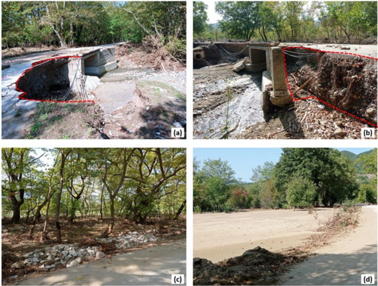
Figure 5.13. Bridge No. 10 crossing a secondary gully on the way from Mouzaki to Ellinokastro (39.401844000° N; 21.668420778° E): (a) western abutment; (b) eastern abutment; and (c) – (d) photos of surrounding fields indicating widespread flooding.
