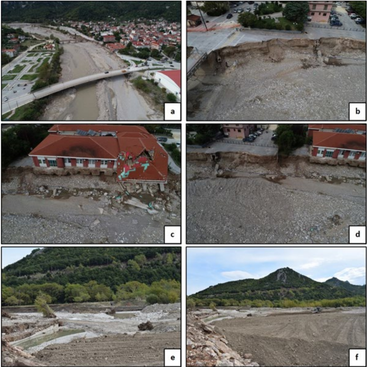
Figure 7.12. Mouzaki road failure (a-d) and remedial measures (e-f) on river embankments (39.427222°N, 21.666667°E).
