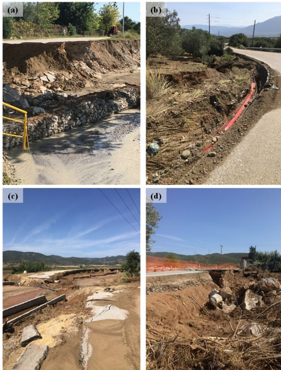
Figure 5.29. Road embankment failures in the region of Lamia: a) at Gorgopotamos (38.83451944°N, 22.39527499°E); b) north of Stirfaka (38.96918055°N, 22.29513611°E); c) along the E.O. Lamia Karpenisi (38.92455°N, 22.27771944°E); d) near Paliouri (38.94233611°N, 22.21619722°E)
