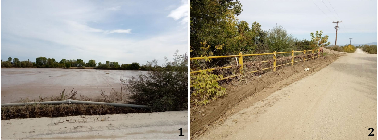
Figure 5.38. 1) Flooded areas south of Megala Kalyvia, Trikala (39.4765°N, 21.7887°E). 2) Road bridge over an irrigation canal (39.4694°N, 21.7907°E). Debris and flood deposits over the deck (upstream view) show that the maximum flood level exceeded the bridge height.
