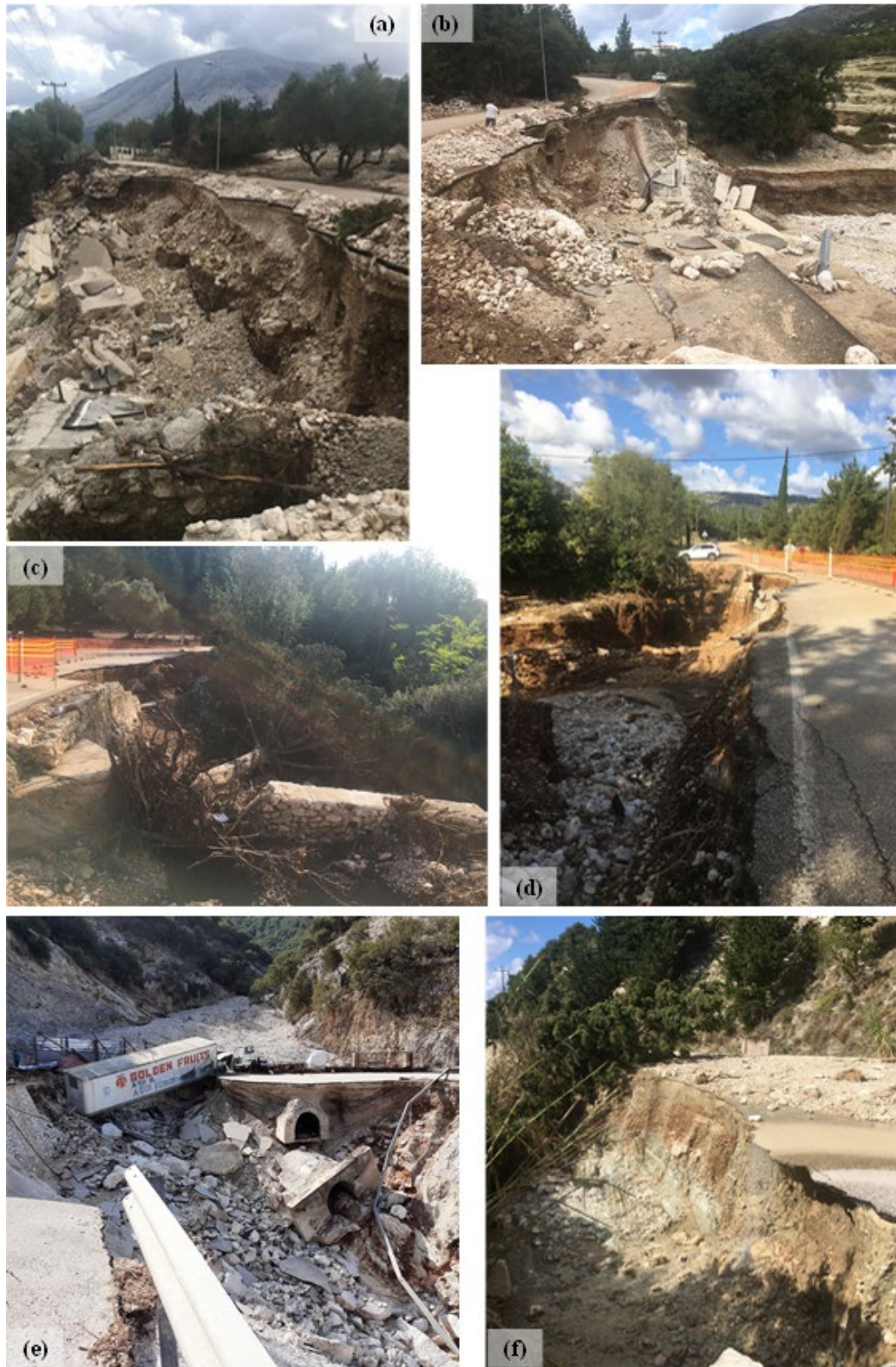
Figure 5.27. Road embankment failures across Cephalonia due to flood/debris related erosion: a,b) 38.325680556°N, 20.551658333°E, c,d) 38.310936111°N, 20.576272222°E, e) 38.326667°N, 20.518333°E, and f) 38.335719444°N, 20.543761111°E
