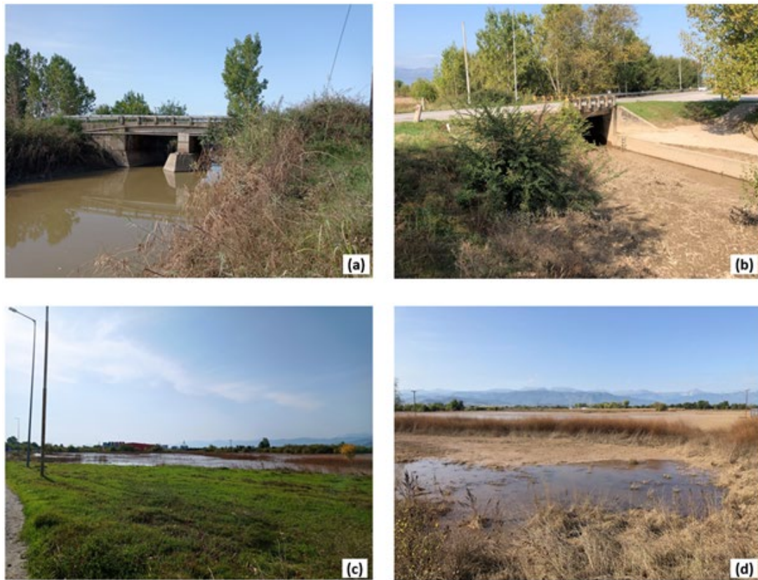
Figure 5.10. Photos of (a) Bridge No.14 (39.097792474°N; 21.878223628°E) and (b) Bridge No. 15 (39.47911111° N; 21.84343611° E) which suffered negligible damage despite being reportedly flooded, with water heights in the (c) – (d) nearby fields exceeding 1.5 m (according to communication with local people).
