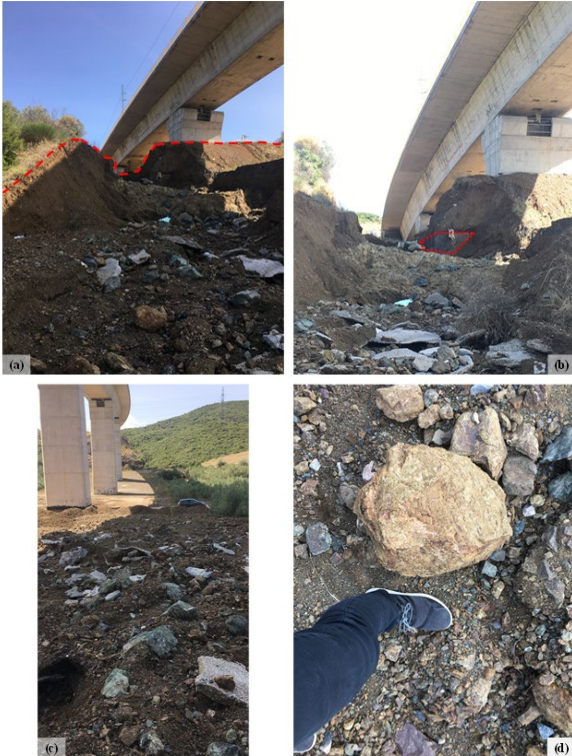
Figure 5.4. Railway bridge foundation scour (38.9609999722°N, 22.3005999722°E): a) eroded scar of bridge foundation embankment, b) exposed pier foundation, c) view of bridge and eroded embankment, and d) indicative size of debris on site
