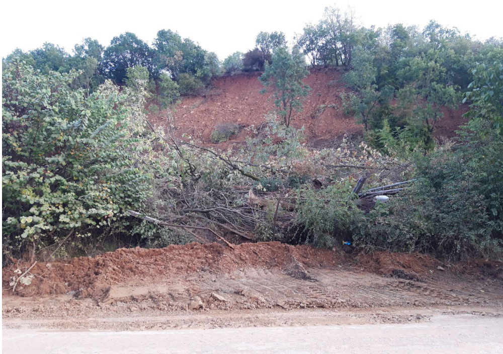
Figure 5.33. Complex rotational-type slope failure near Rachoula (39.2494490°N, 21.8889110°E)
