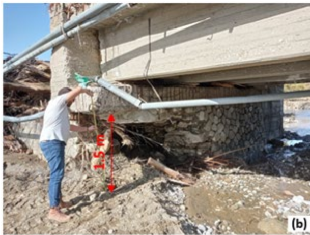
Figure 5.14. Photos of Bridge No. 13 located east of the Plastiras lake ( 39.309563356^{\circ}\text{N} ; 21.710816055^{\circ}\text{E} ): (a) side view indicating debris built-up and (b) significant abutment scouring and (c) backfill erosion that leads to the partial collapse of the roadway.
