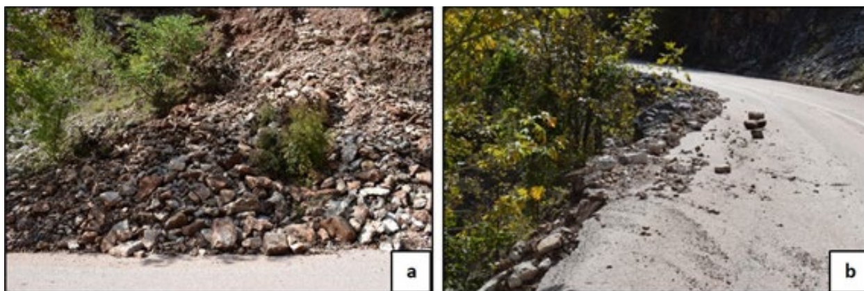
Figure 6.31. Rockslide along the road from Argithea to Zervo village road (39.348333°N, 21.517222°E)
