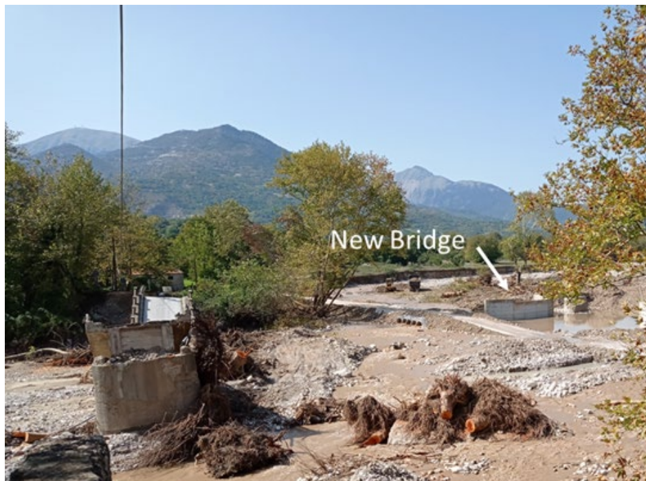
Figure 5.23. New bridge being constructed next to the collapsed bridge No. 11.
