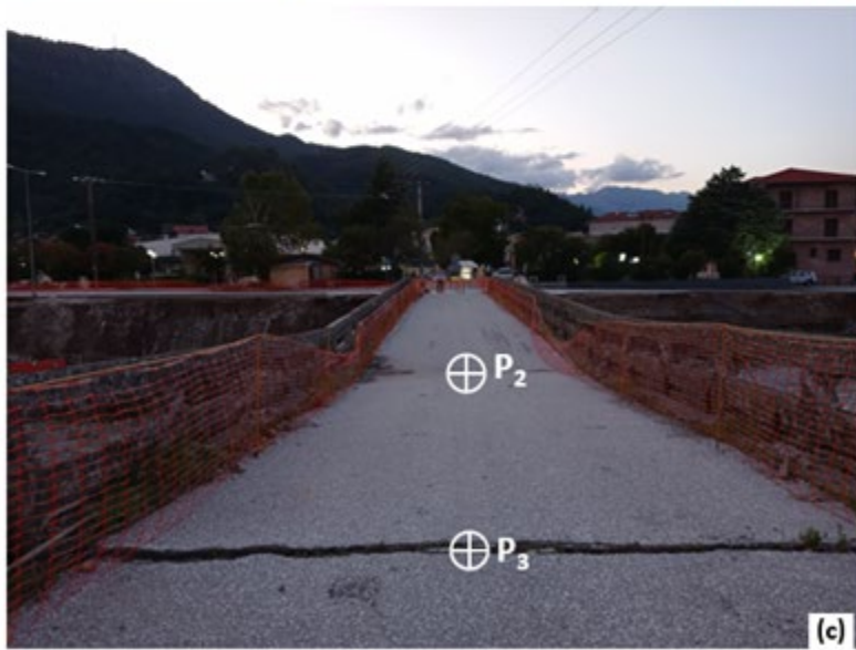
Figure 5.18. Photos of Bridge No. 8 taken from the level of the roadway: (a) abutment erosion; (b) settlement induced step; (c) – (d) extension cracks over Pier 3.
