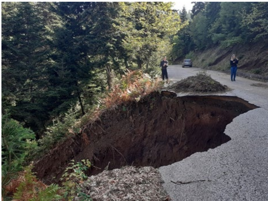
Figure 6.20. Rotational slide in weathered mantle that caused damage to road (39.2174890°N, 21.7949870°E)
