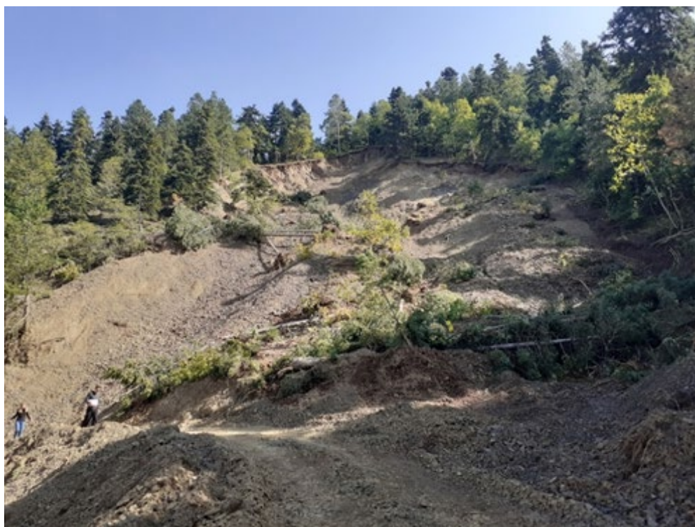
Figure 6.7. Complex slide (rotational and earth slide) in shale dominant flysch. The slipped material has completely covered the road (39.2116910°N, 21.7942940°E)
