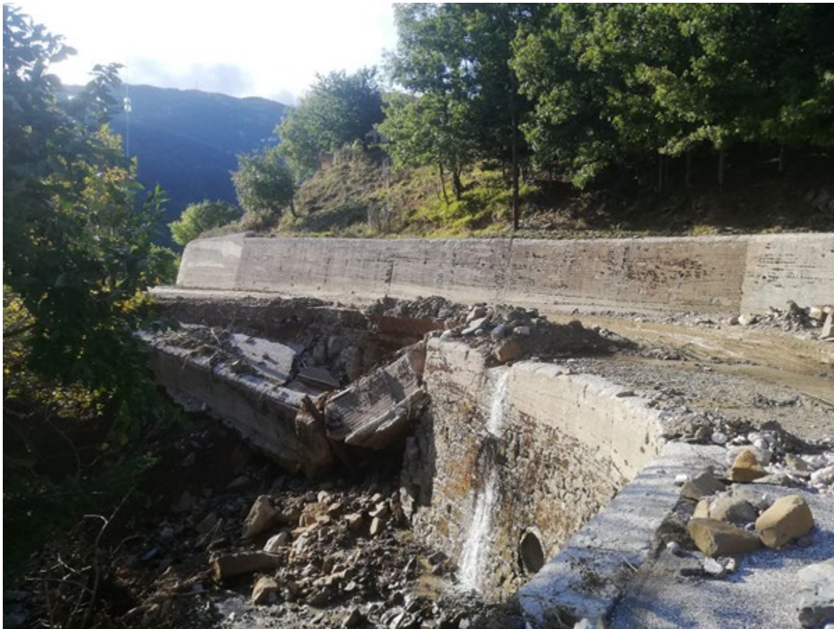
Figure 7.20. Riverbank erosion – slope failure that damaged partially the road. (39.26247°N, 21.71319°E)
