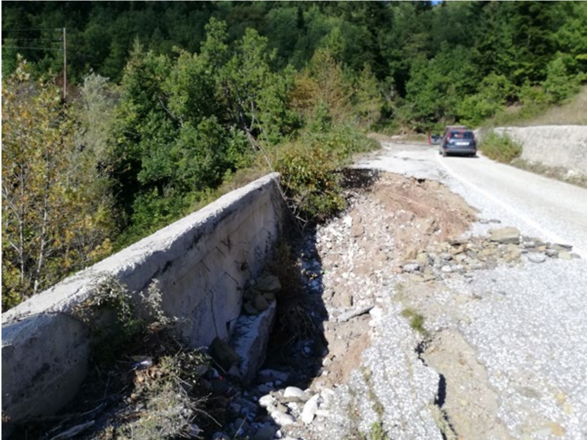
Figure 7.23. Extensive surface erosion on the side of Belokomiti - Karditsa road. (39.26022°N, 21.72556°E).
