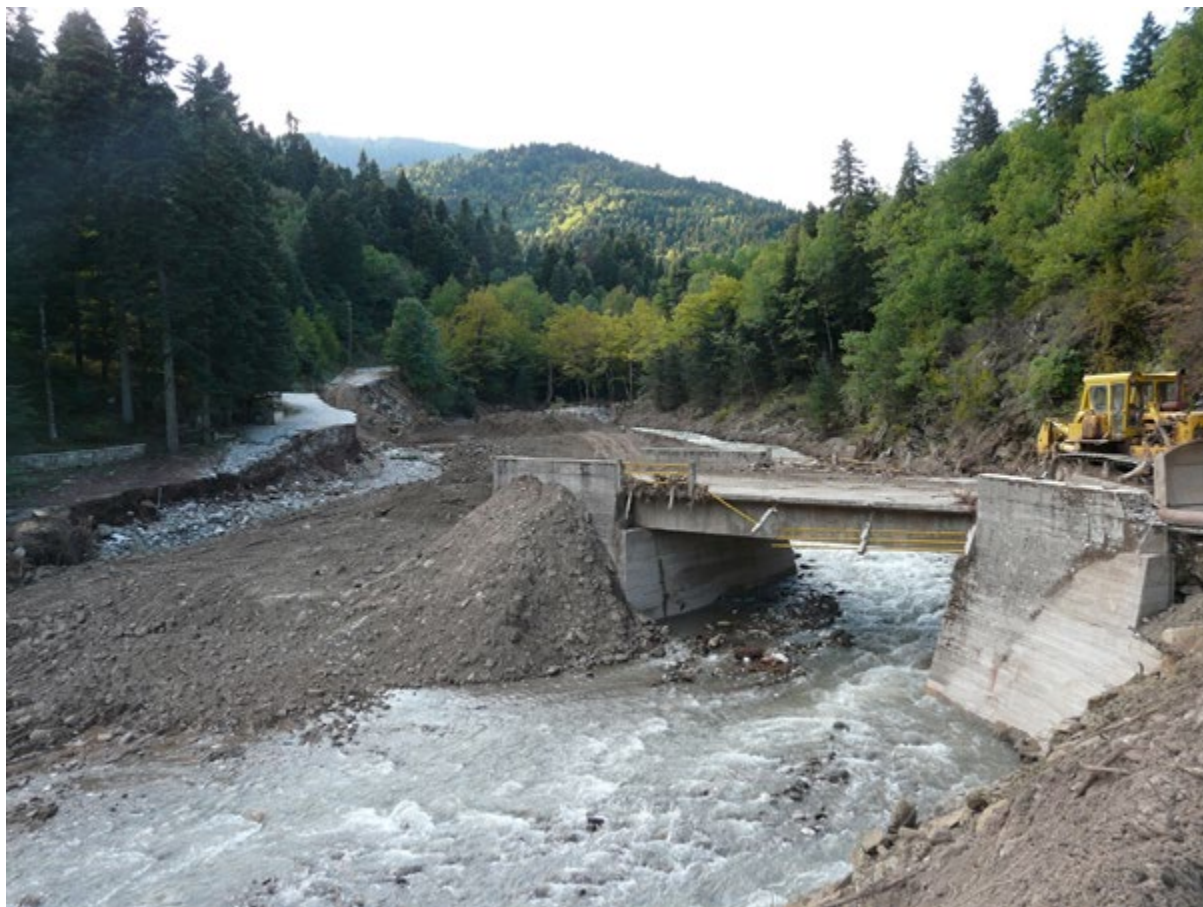
Figure 7.15. Riverbank erosion – slope failure that blocked the road. Karitsiotis river bridge, south of Belokomiti, Plastira Lake. (39.25381°N, 21.71591°E).
