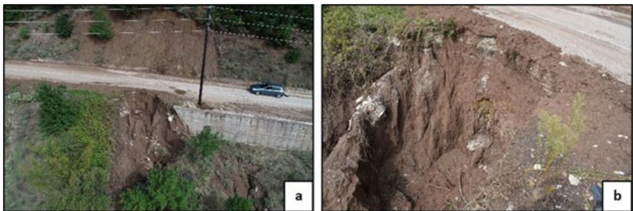
Figure 6.16. Rotational slide towards Porti village (39.425833°N, 21.665556°E)
