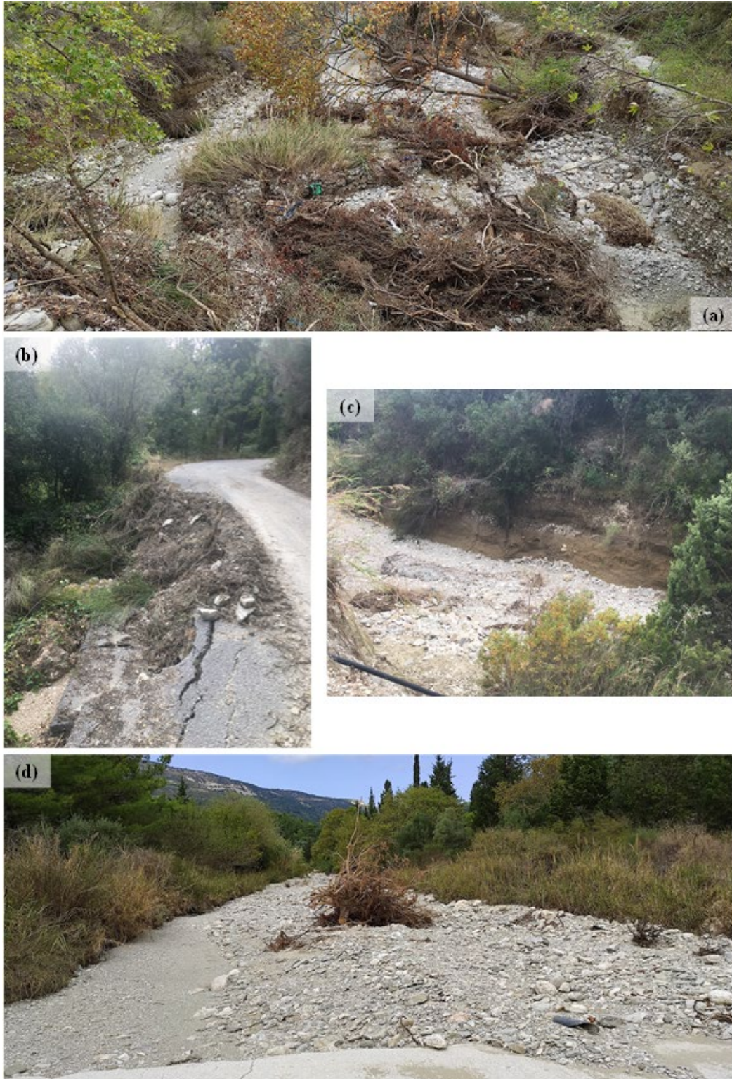
Figure 7.4. Typical features observed in Lefkada island: a) eroded material from flood protection levee (38.665858972°N, 20.620208°E); b) road embankment damage (38.67684167°N, 20.6093056°E); c) riverbank erosion (38.6646278°N, 20.623711°E); d) debris on riverbed (38.665858972°N, 20.620208°E).
