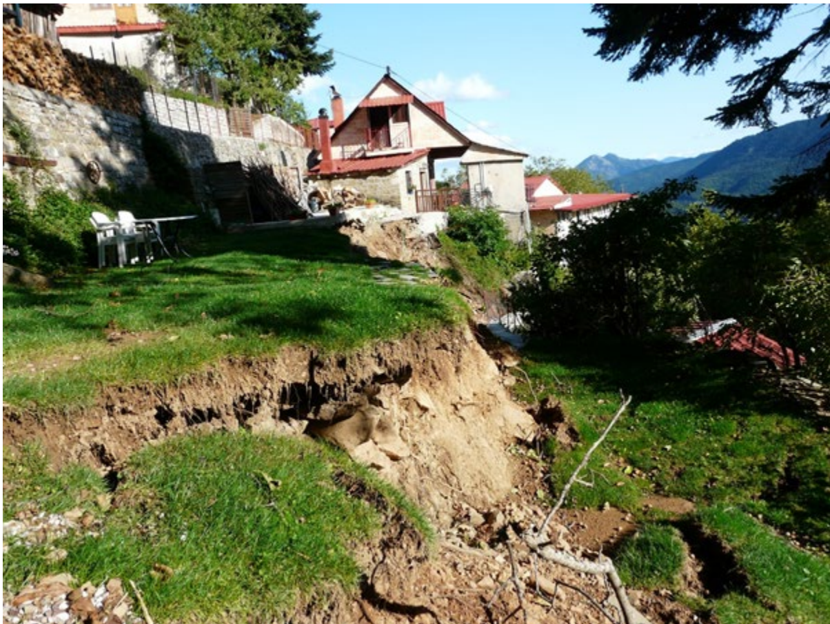
Figure 6.18. Rotational slide causing structural damage at the village of Rafina (39.27172°N, 21.69607° E)
