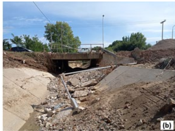
Figure 5.8. Photos of Bridge No. 5 (39.346522222°N; 21.920672222°E): (a) debris has been moved to the side; (b) debris built up in front of the neighboring overpass of the irrigation trench.
