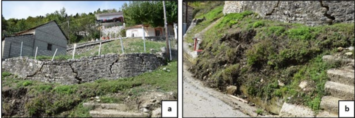
Figure 6.17. Rotational slide on the road to Oxya village that damaged a retaining wall (39.358889°N, 21.596111°E)
