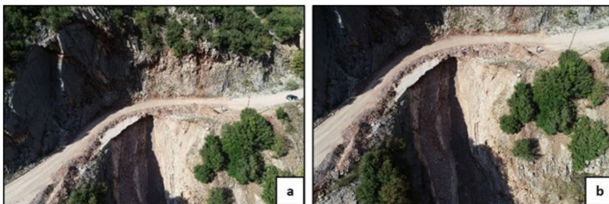
Figure 6.32. Rockslide along the Argithea to Zervo road network (39.354167°N, 21.5175°E).
