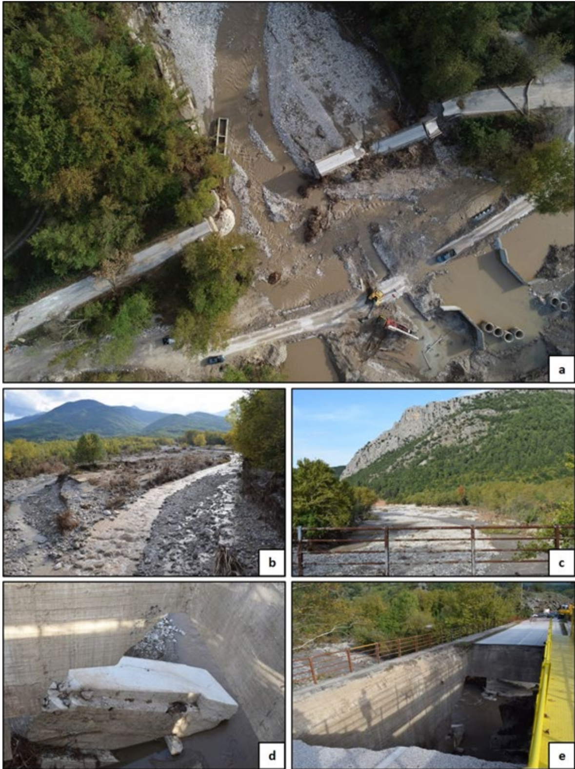
Figure 7.13. Debris flow caused damage to the bridges of a) Karaiskakis (39.401667 N, 21.653333 E), and b-e) Mpalanos (39.406111°N, 21.662778°E).
