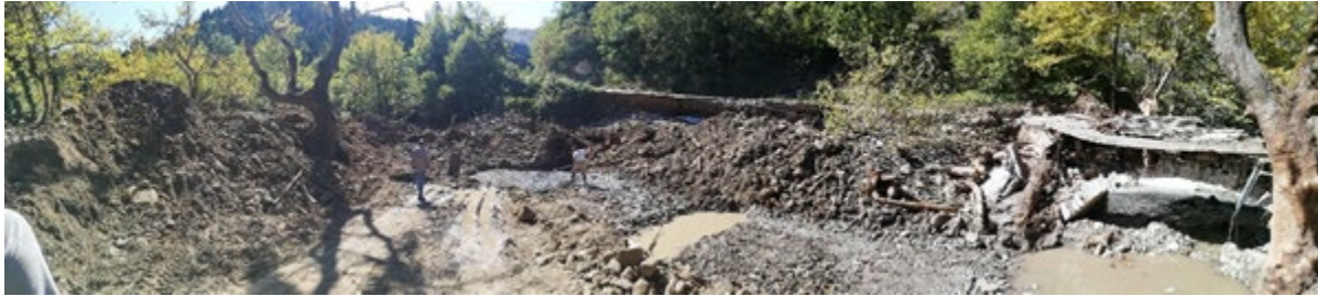
Figure 7.19. Riverbank erosion – slope failure that damaged the road at the village Pezoula. (39.30351°N, 21.6876°E)
