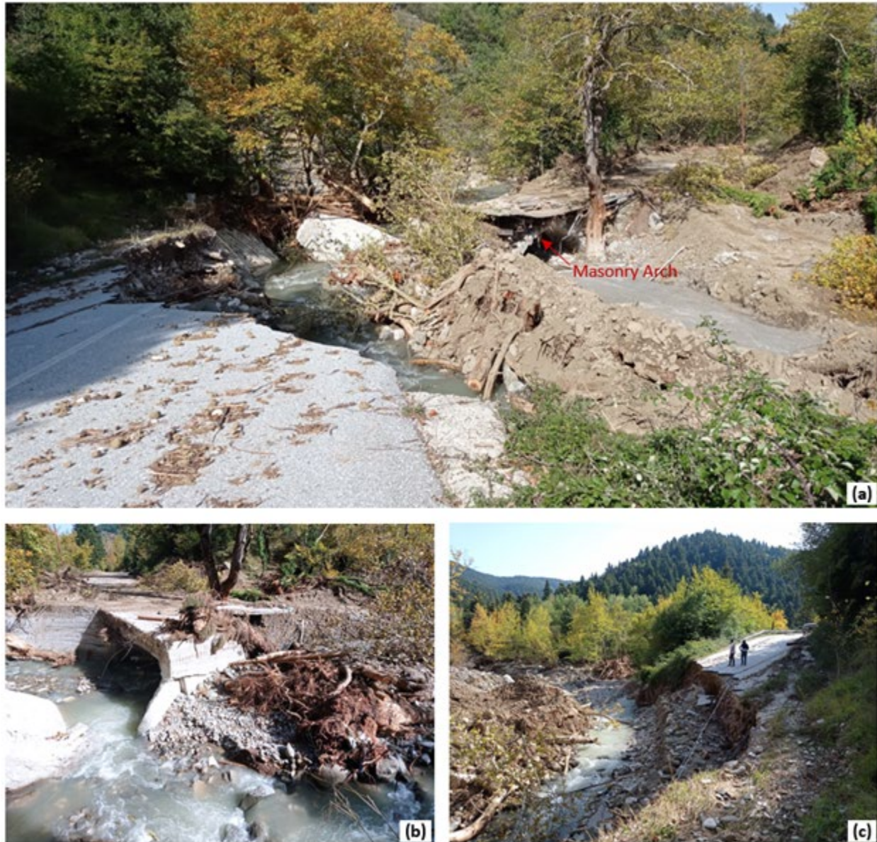
Figure 5.26. Photos of Bridge No.12, a masonry arch located on the way from Filakti to Pezoula ( 39.303508426^{\circ}\text{N} ; 21.686573208^{\circ}\text{E} ): (a) – (b) suffering extended abutment and riverside erosion that lead to (c) collapse of the roadway.
