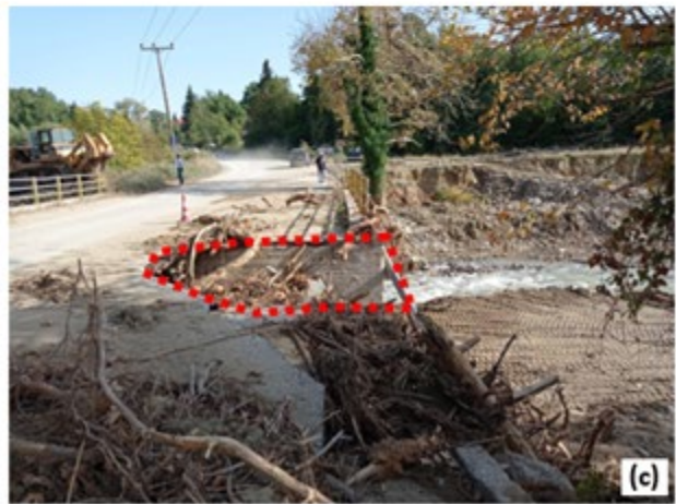
Figure 5.14. Photos of Bridge No. 13 located east of the Plastiras lake ( 39.309563356^{\circ}\text{N} ; 21.710816055^{\circ}\text{E} ): (a) side view indicating debris built-up and (b) significant abutment scouring and (c) backfill erosion that leads to the partial collapse of the roadway.
