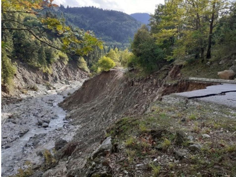
Figure 7.24. Riverbank erosion – slope failure that totally damaged the road at Vlasi village (39.2906260°N, 21.5862230°E).
