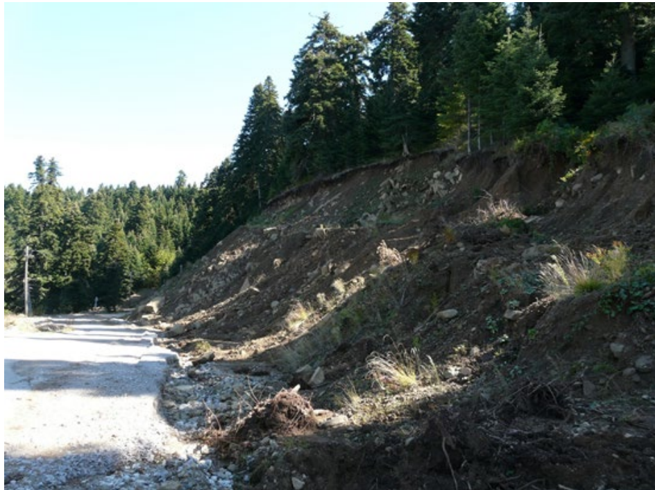
Figure 6.19. Rotational slide inducing damage on the road network (39.28596°N, 21.69099° E)
