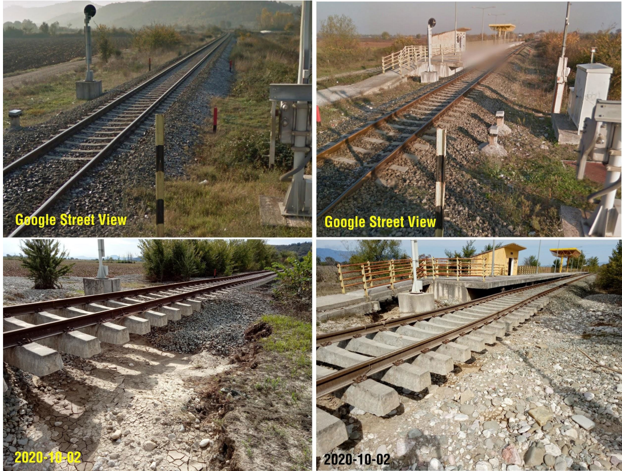
Figure 5.42. Railway embankment & ballast scouring along Paleofarsalos-Kalabaka line, Magoula station (39.45127°N, 21.78824°E). Comparison of field photo (bottom) with pre-event Google Street View image (top).
