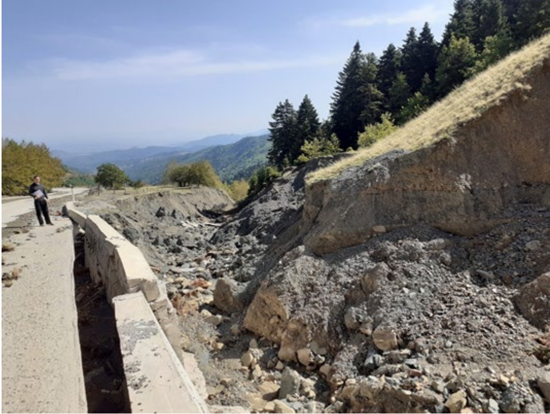
Figure 7.26. Extensive surface erosion on the side of Kastania – Rachoula road. Failure of retaining wall (39.2314830°N, 21.8016040°E).
