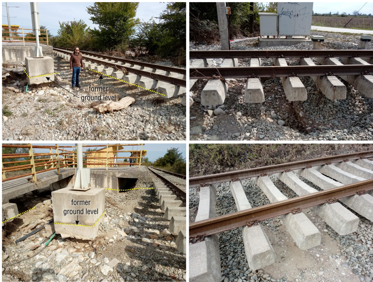
Figure 5.40. Railway embankment & ballast scouring at Magoula train station (39.45127°N, 21.78824°E).
