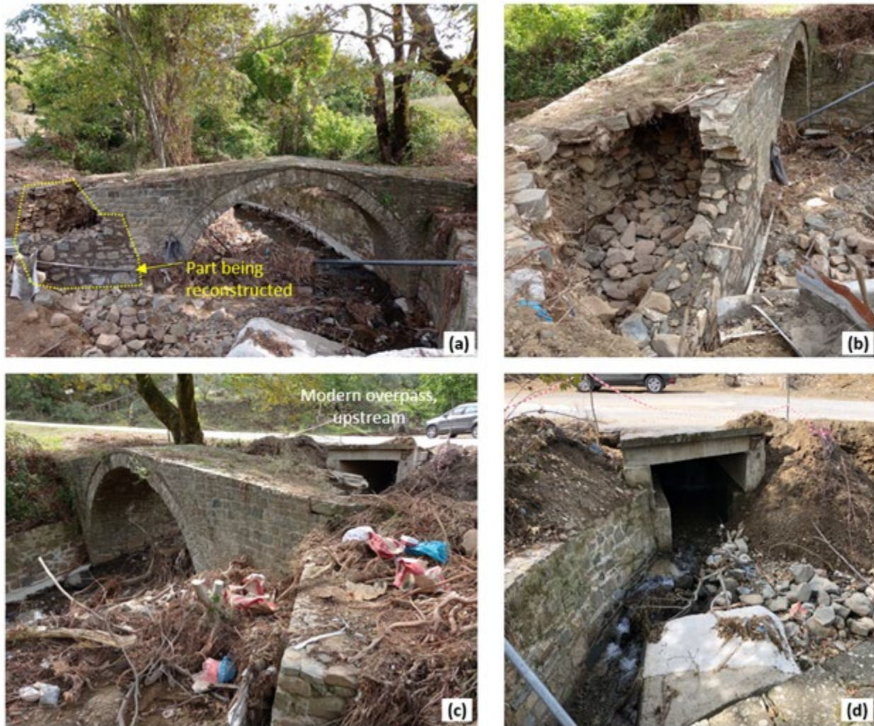
Figure 5.25. Photos of Bridge No.2, a masonry arch near Moschato (39.32248333°N; 21.79625000°E): (a) – (b) part of it was being reconstructed on 2/10/2020, while (c) there was a significant amount of debris upstream, especially in the (d) modern (RC) overpass.
