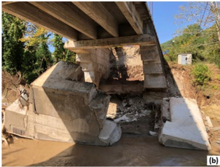
Figure 5.12. Photos of the collapsed Bridge No. 9 crossing Pamisos river about 2 km north of Mouzaki ( 39.406108333^{\circ}\text{N} ; 21.663150000^{\circ}\text{E} ): (a) side view indicating abutment backfill erosion and the location of the collapsed roadway segment; (b) closer view of failed abutment wall; and (c) the roadway gap.
