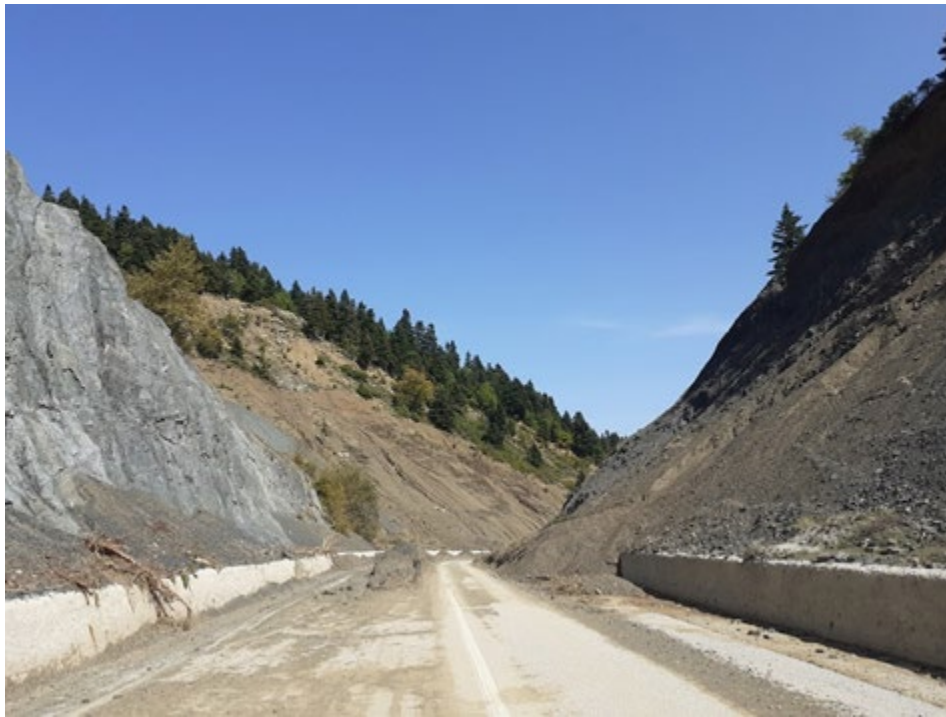
Figure 5.31. Landslips from side slopes along the Kastania – Rachoula section (39.2314830°N, 21.8016040°E)
