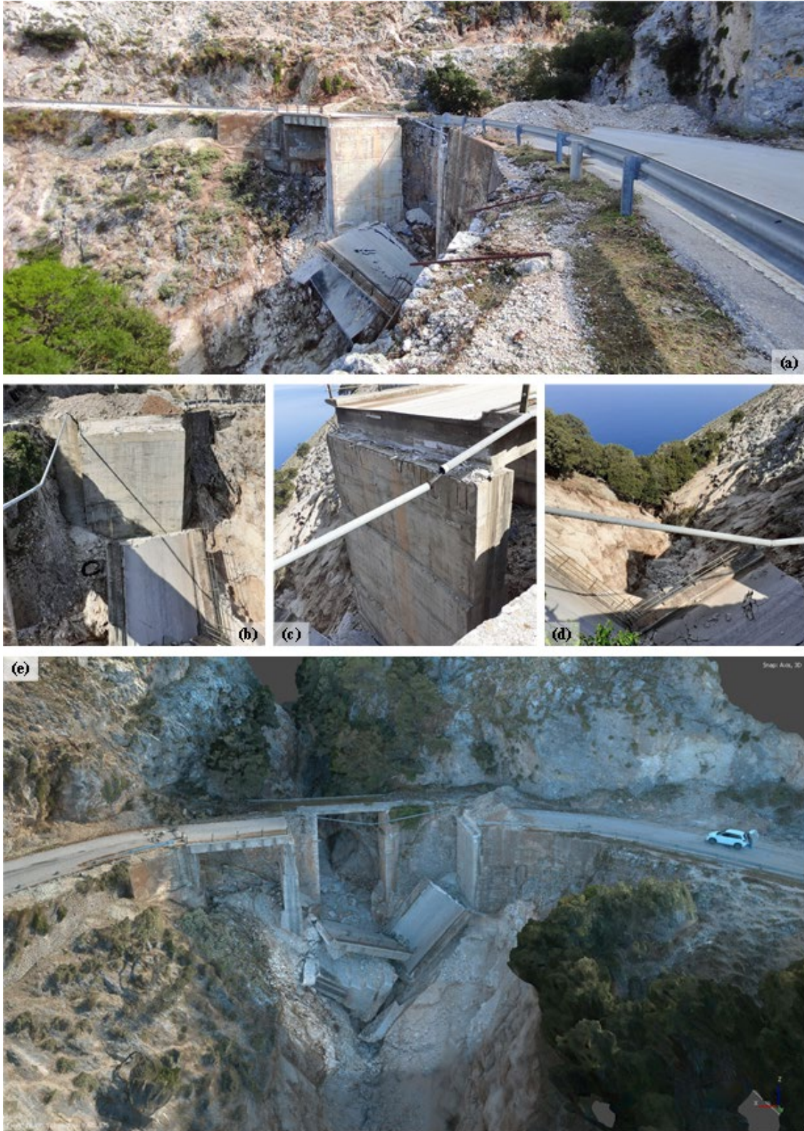
Figure 5.1. Collapsed multi-span RC bridge on E.O. Argostoliou-Fiskardou ( 38.319506^{\circ}\text{N} , 20.508197^{\circ}\text{E} ): a-d) roadside photos, e) UAV-enabled 3D texture mesh - perspective view (view 3D model at: https://skfb.ly/6WyYT )
