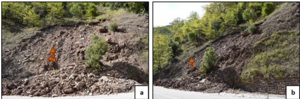
Figure 6.9. Rotational slide along the Argithea to Zervo village road (39.351111°N, 21.521389°)
