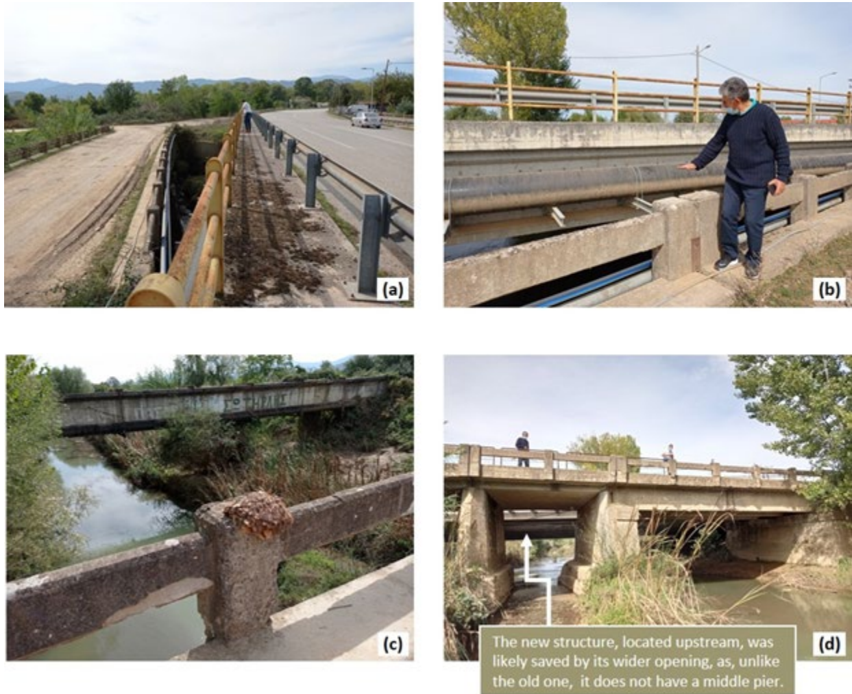
Figure 5.6. Photos of Bridge No. 3: a pair of RC bridges crossing the Gavria Rema along the Karditsa – Kastania provincial road (39.344589222°N; 21.894189833°E): (a) evidence of overflow over the older bridge, which is located a few meters downstream of the younger structure; (b) level of water height; (c) debris remains at the deck; and (d) side view of the structure showing no structural damage.
