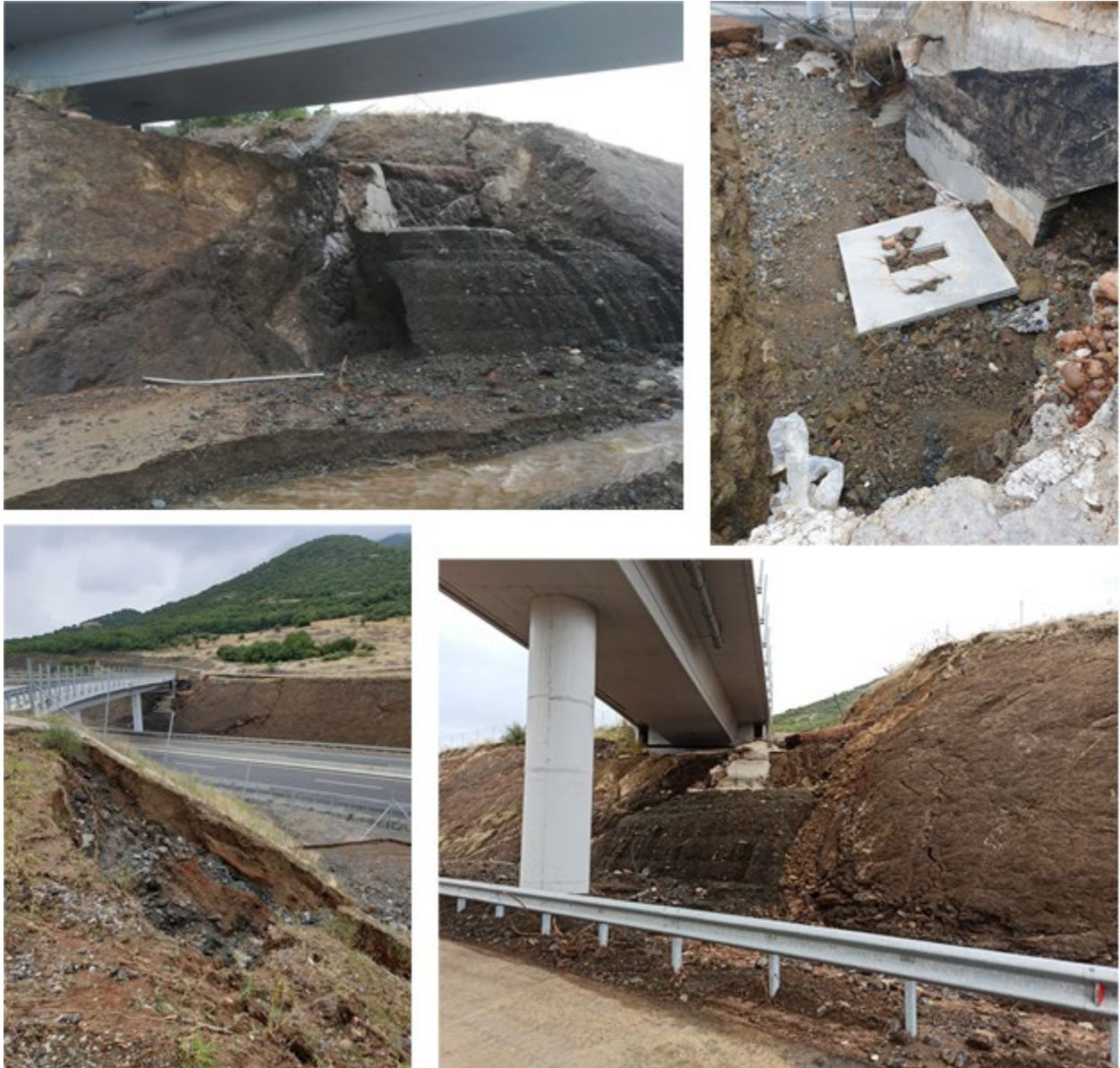
Figure 7.11. Bridge embankment erosion on Highway E65, km+56 outside the town of Anavra (39.172474°N, 22.091382°E) (view 3D model at: https://skfb.ly/6W7AK ).
