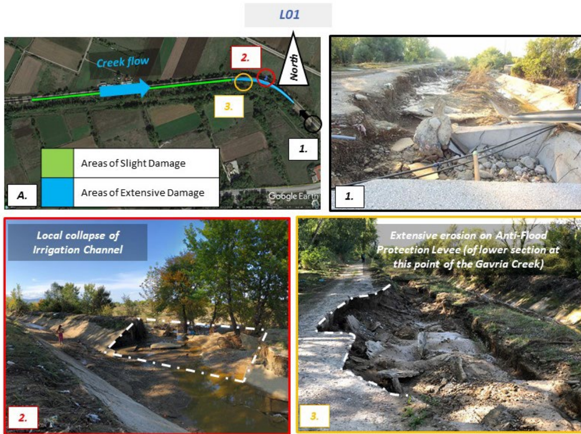
Figure 8.6. (A) location of Flood Protection Levee 01 ( 39.347550^{\circ}\text{N} ; 21.890664^{\circ}\text{E} ) – the Flood Protection Levee sustained extensive damages over an area of \sim 2,500 \text{ m}^2 (light blue) and slight damage over an area of \sim 5,500 \text{ m}^2 (light green); (1) extensive damage with bottom-up erosion of the levee (courtesy of Mr. Apostolos Vergis ); (2) local collapse of the irrigation channel section, (3) extensive erosion of the levee downstream the irrigation channel failure.
