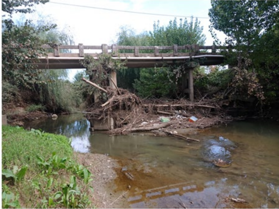
Figure 5.7. Photos of Bridge No. 4 of the Gavria Rema (39.348575°N; 21.904591667°E) showing significant debris build-up, but no other damage.
