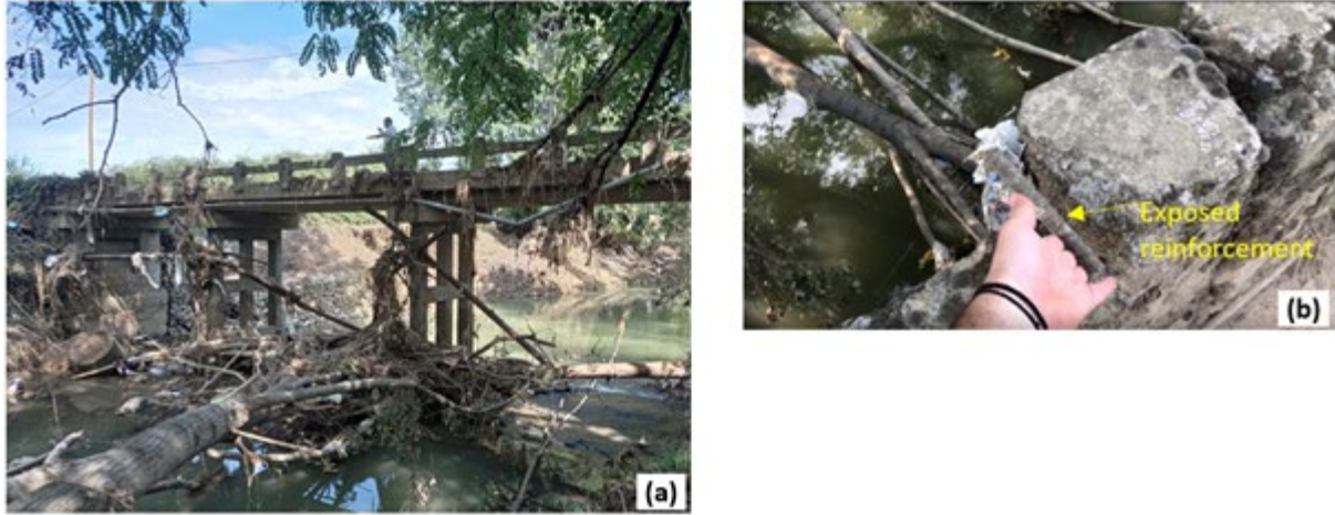
Figure 5.9. Photos of Bridge No.6 (39.344589222°N; 21.894189833°E): (a) debris has been moved to the side; (b) no evidence of flood induced damage despite the bridge being old and poorly maintained with exposed reinforcement.
