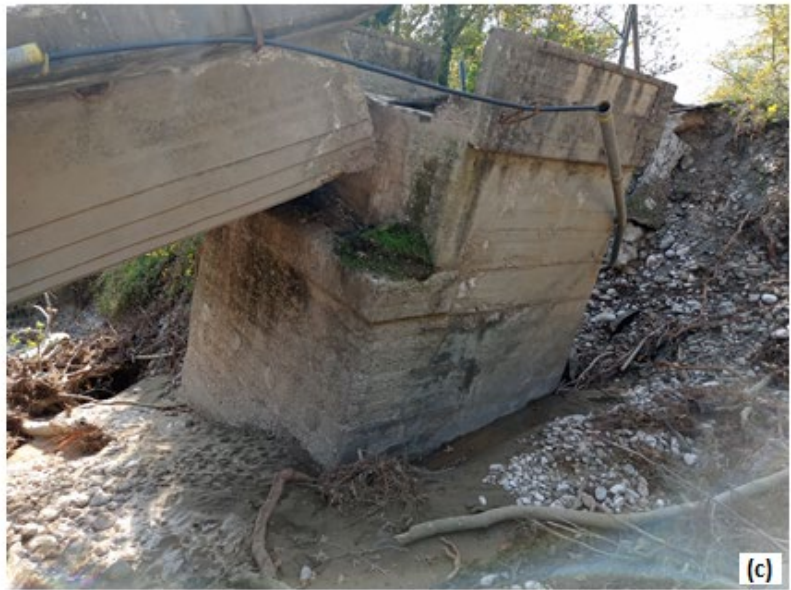
Figure 5.21. Photos of Bridge No. 11 ( 39.401172611^{\circ}\text{N} ; 21.652868250^{\circ}\text{E} ) which evidently collapsed due to a combination of abutment and pier scour: (a) side view, (b) - (c) bearing capacity failure of the abutment and deck collapse.
