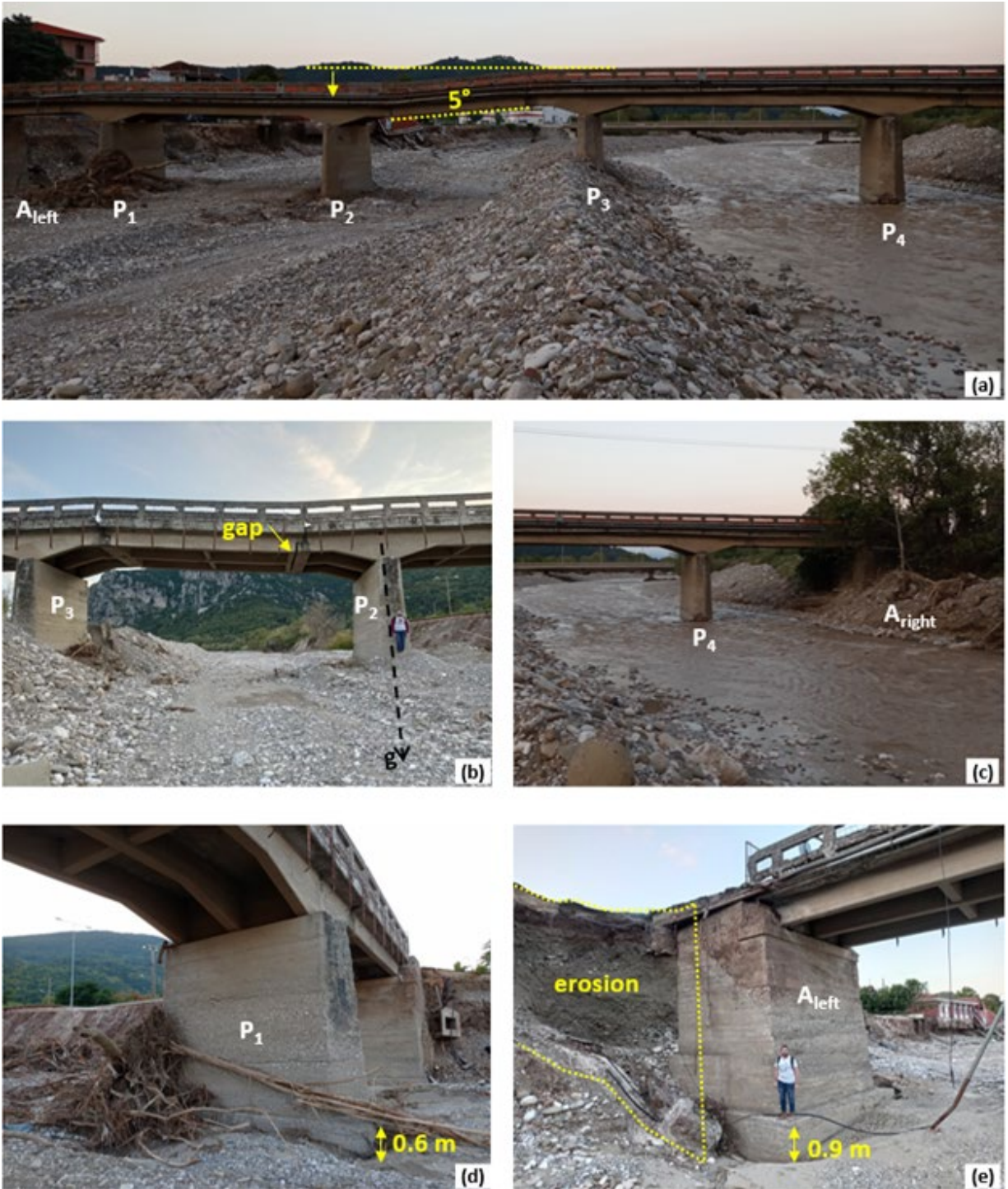
Figure 5.17. Photos of the severely damaged pedestrian bridge in Mouzaki, i.e. Bridge No. 8 (39.425804111°N; 21.666233056°E): (a) longitudinal direction indicating the substantial settlement of the left side (Pier 2) and the associated rotation of the deck; (b) closer view of piers 2 and 3; (c) the evidently unaffected right side; (d) scour at P1; and (e) abutment scour and backfill erosion.
