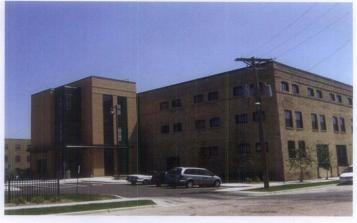
Figure 8. The rehabilitation of this large, early-20th century warehouse (left) into affordable artists' lofts included the addition of a compatible glass and brick elevator/stair tower at the back (right).
