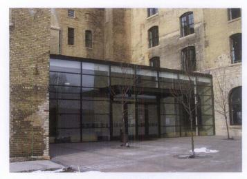
Figure 14. This glass addition was erected at the back of an 1895 former brewery during rehabilitation to provide another entrance. The addition is compatible with the plain character of this secondary elevation.
