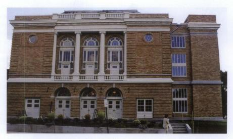
Figure 7. A vacant side lot was the only place a new stair tower could be built when this 1903 theater was rehabilitated as a performing arts center. Constructed with matching materials, the stair tower is set back with a recessed connector and, despite its prominent location, it is clearly subordinate and differentiated from the historic theater.
