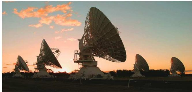
FIG. A.9. Five of the six identical Cassegrain antennae that comprise the *ATCA* (Wilson et al., 2011).
