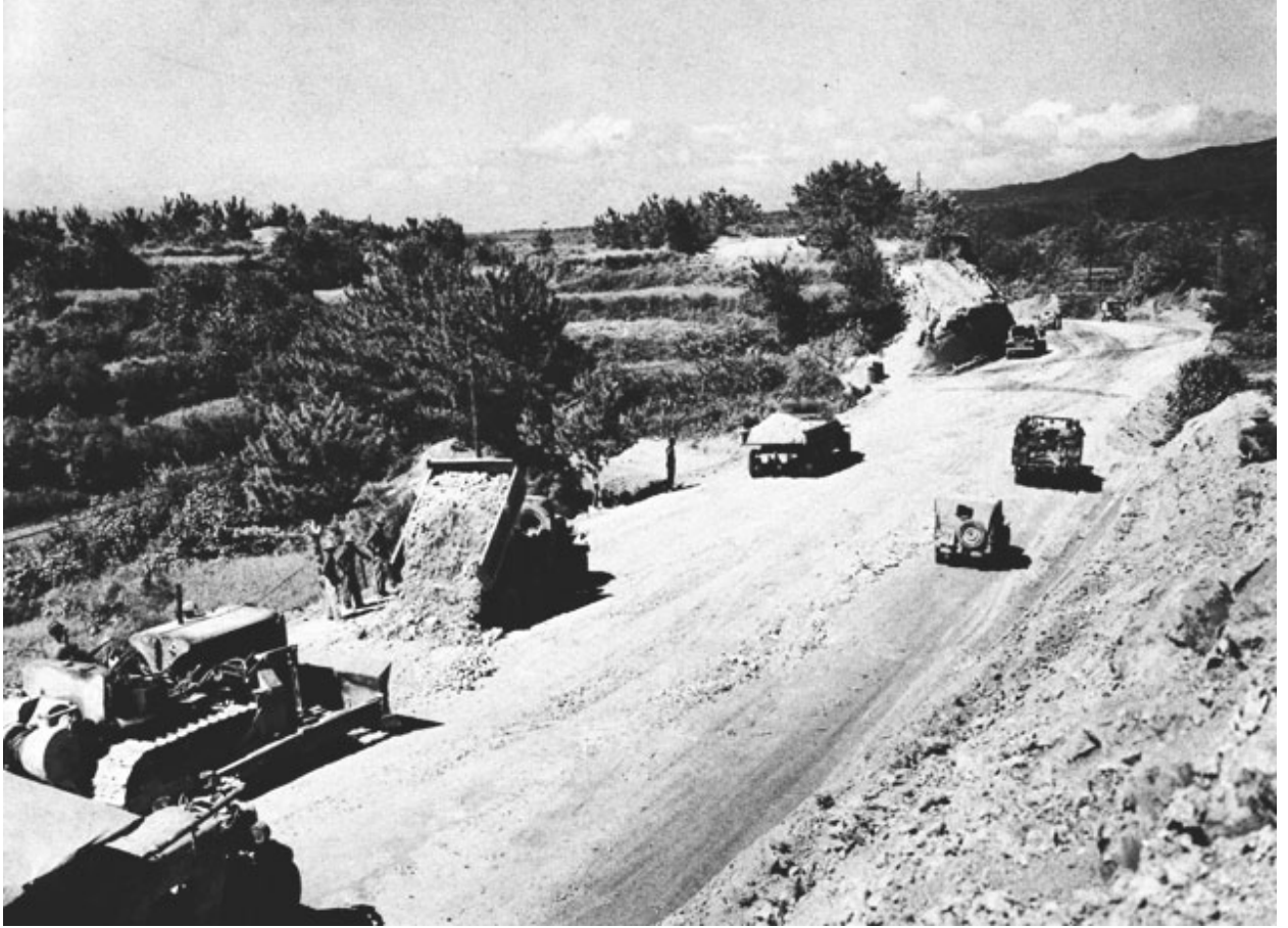
Figure 12. Road-Surfacing Operations by the 71st Seabees on Okinawa, 1945. https://www.ibiblio.org/hyperwar/USN/Building_Bases/bases-30.html .
