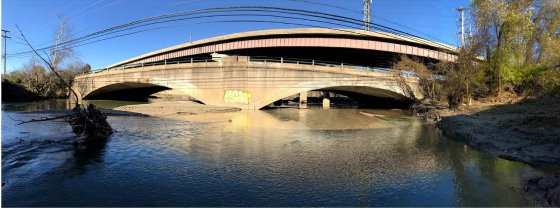
*Image 1.1: [Facing upstream] The Route 1 culvert that bisects the study area into two sections is split into two arches. Sediment regularly collects underneath the arches, to be later flushed out by high velocity flow during storm events. Credit for images: Zach Clifton*
