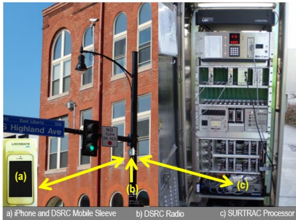
Figure 2-2: Schematic of Different Elements of the Safe Intersection Crossing Application
